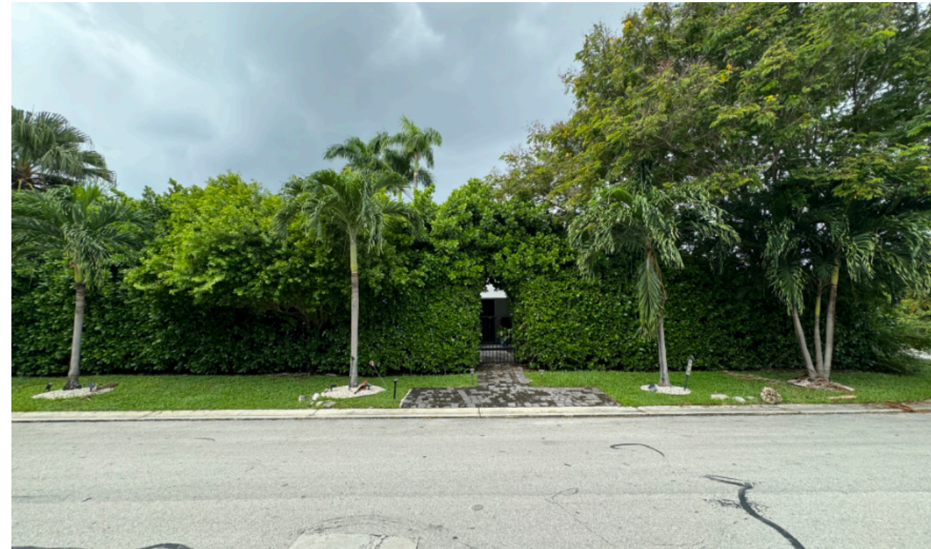
10 322 E. DI LIDO DRIVE EXISTING ONE-STORY RESIDENCE
