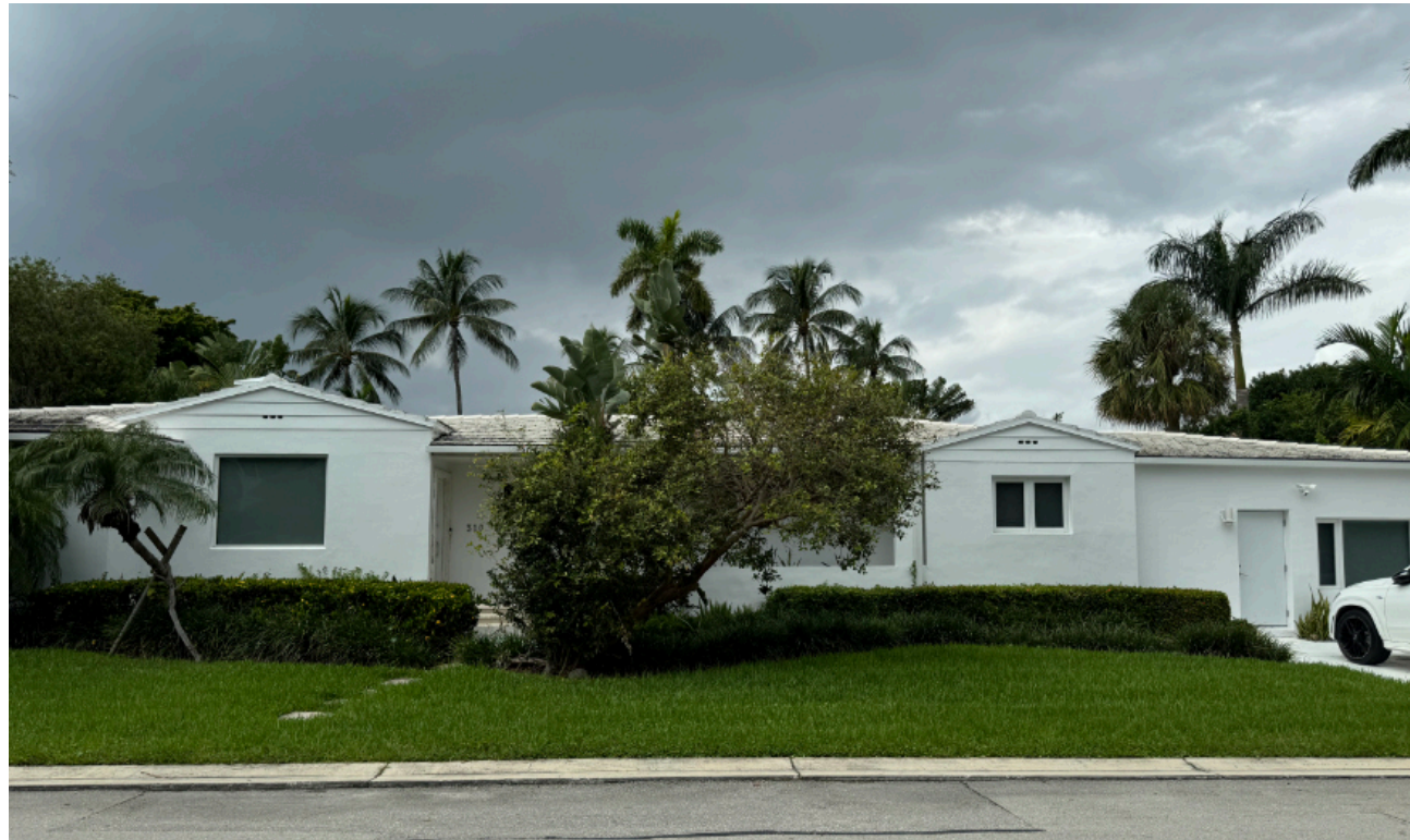
9 310 E. DI LIDO DRIVE EXISTING ONE-STORY RESIDENCE
