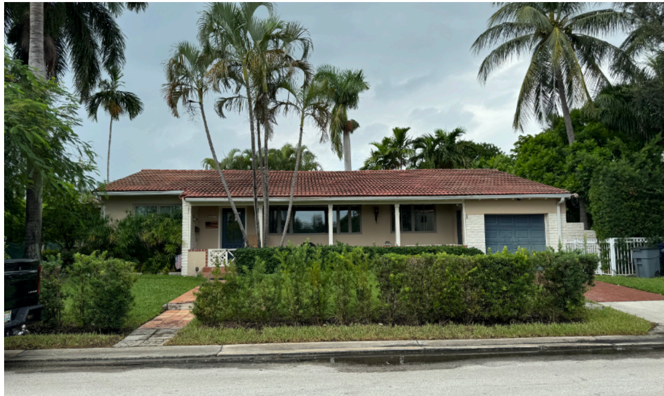
11 400 E. DI LIDO DRIVE EXISTING ONE-STORY RESIDENCE
