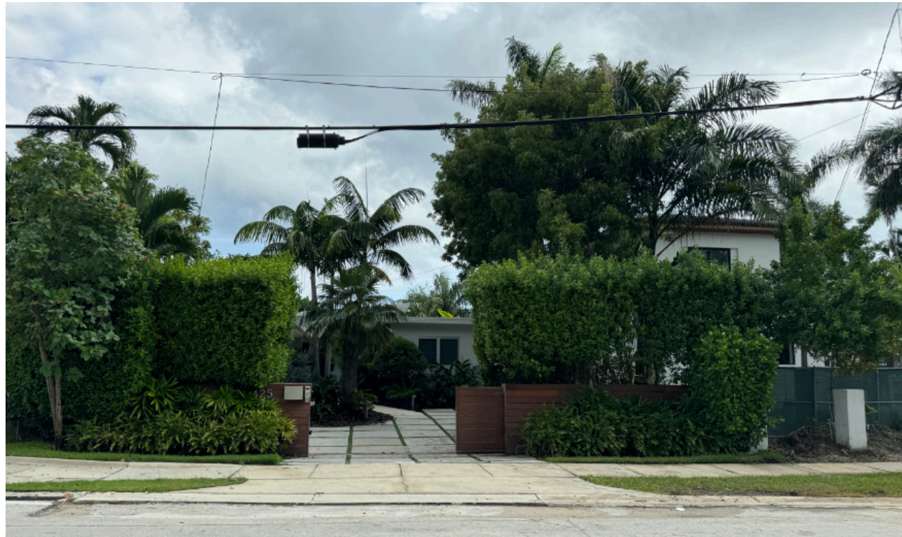
1 425 E. DI LIDO DRIVE EXISTING ONE-STORY RESIDENCE
