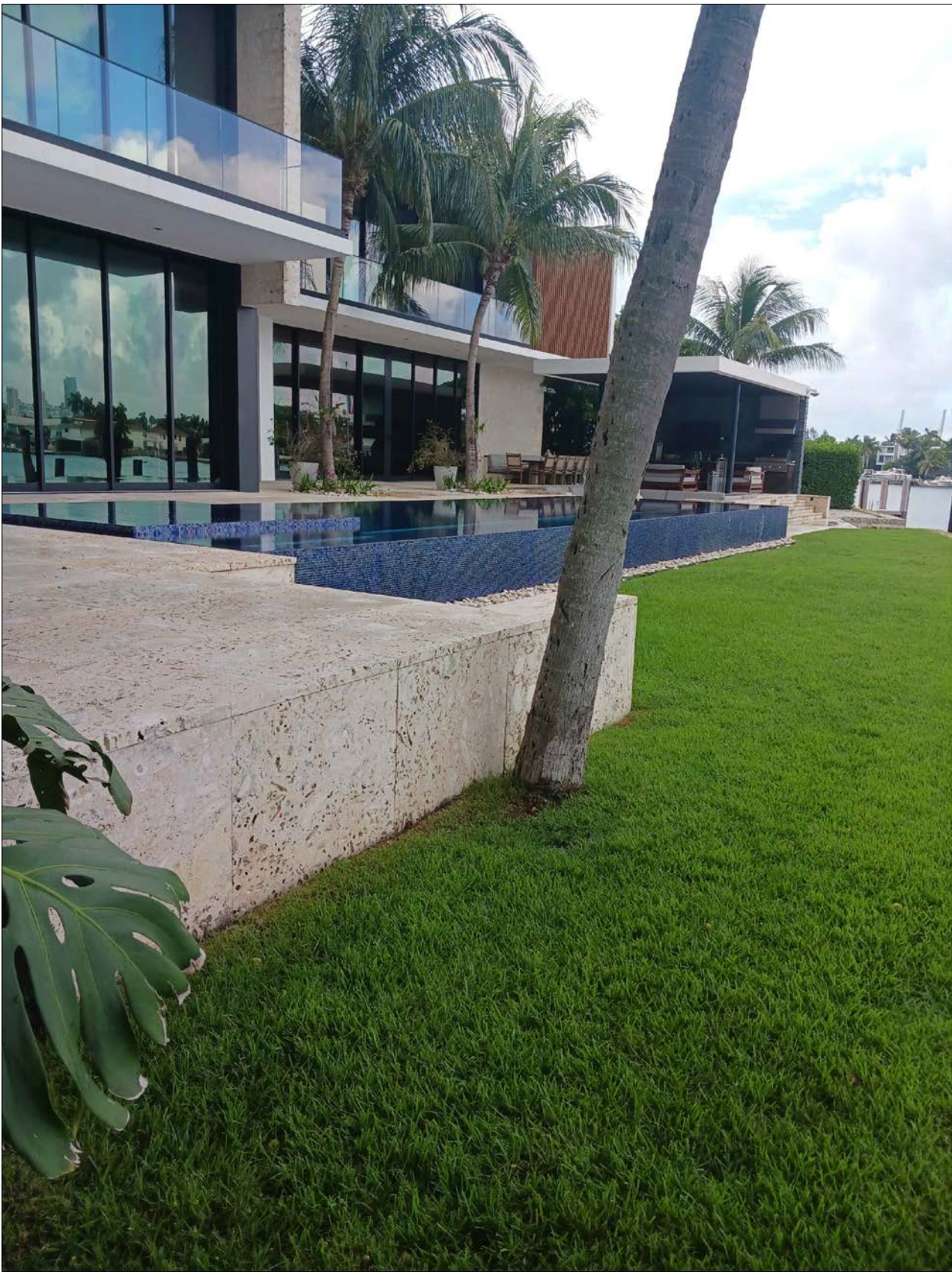
② REAR LOOKING NORTHEAST
