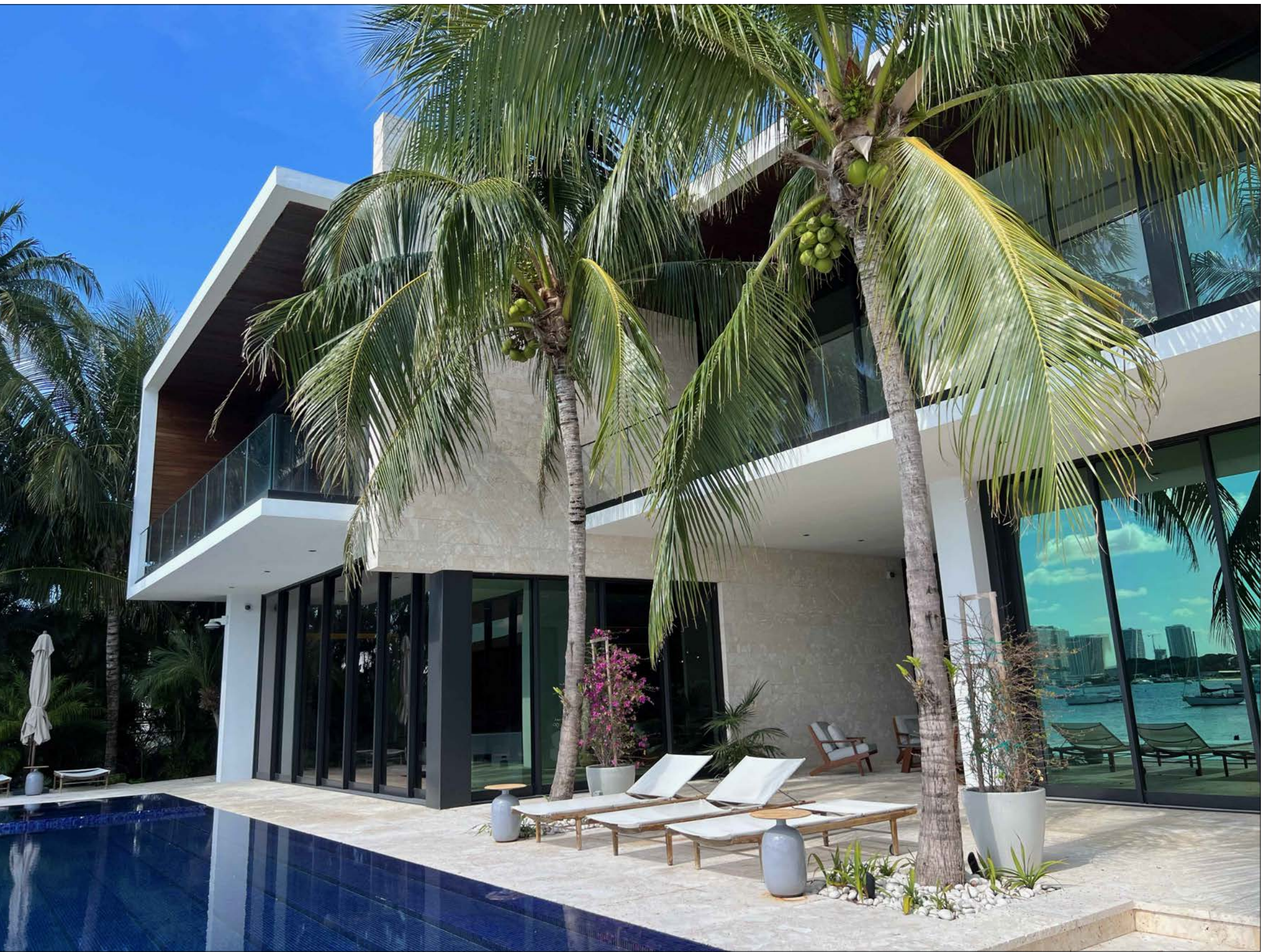
④ REAR - LOOKING NORTHWEST
