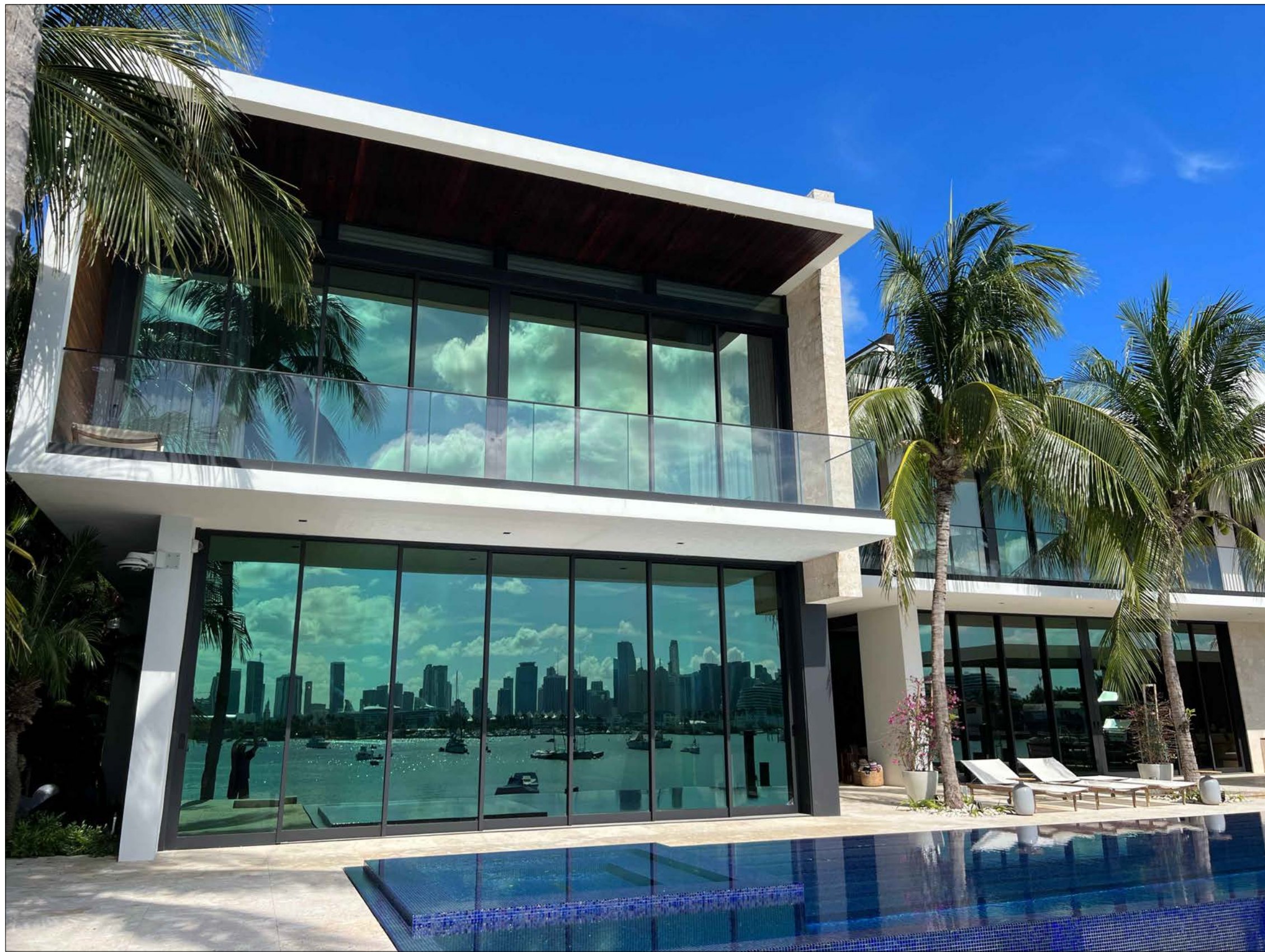
③ REAR LOOKING NORTH
