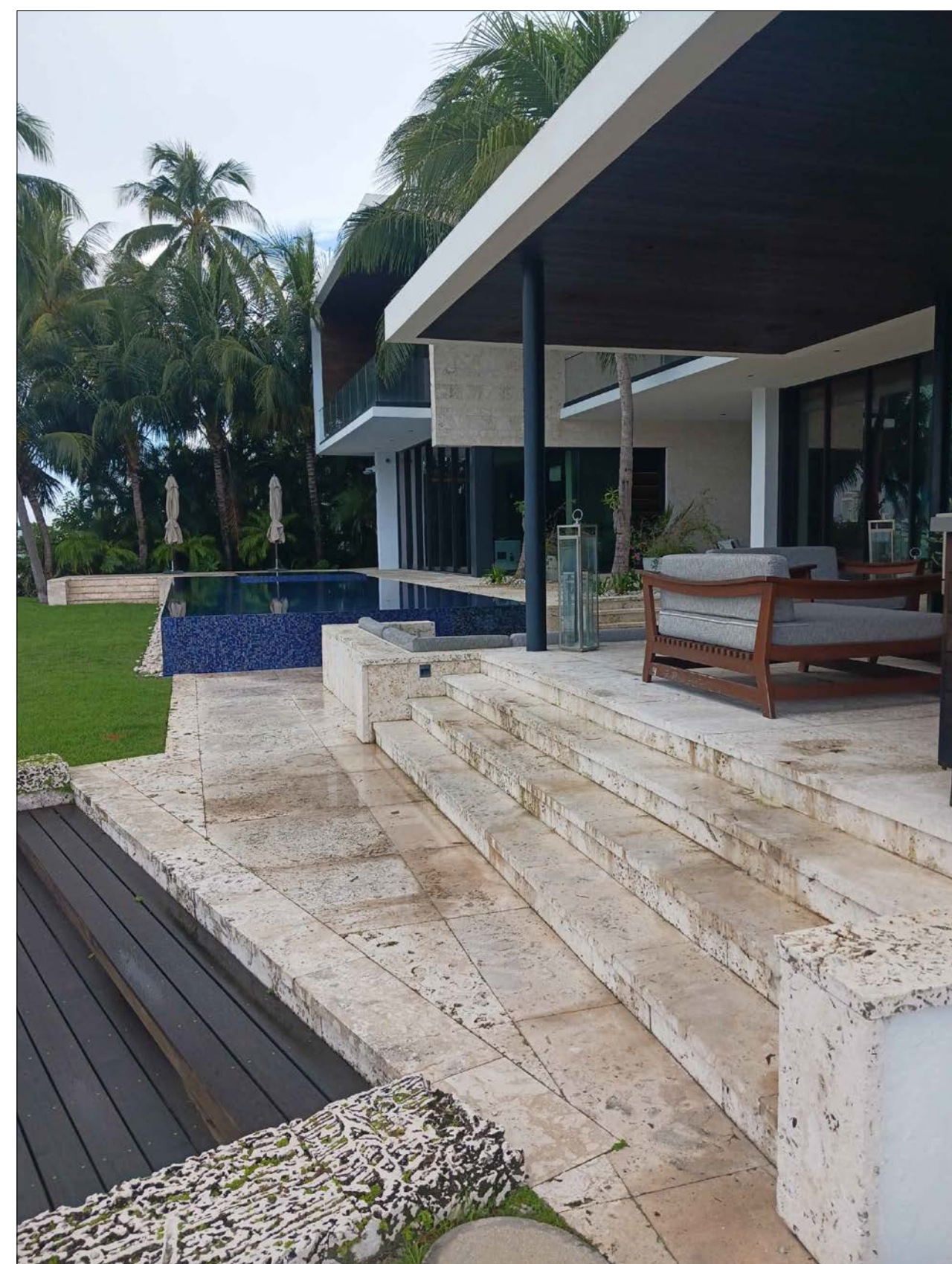
① REAR LOOKING NORTHWEST
