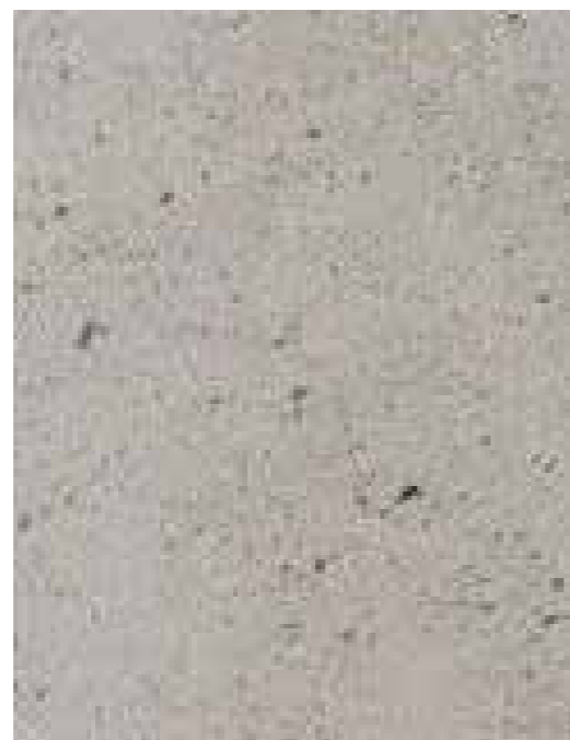
Exterior face of ramp - concrete
