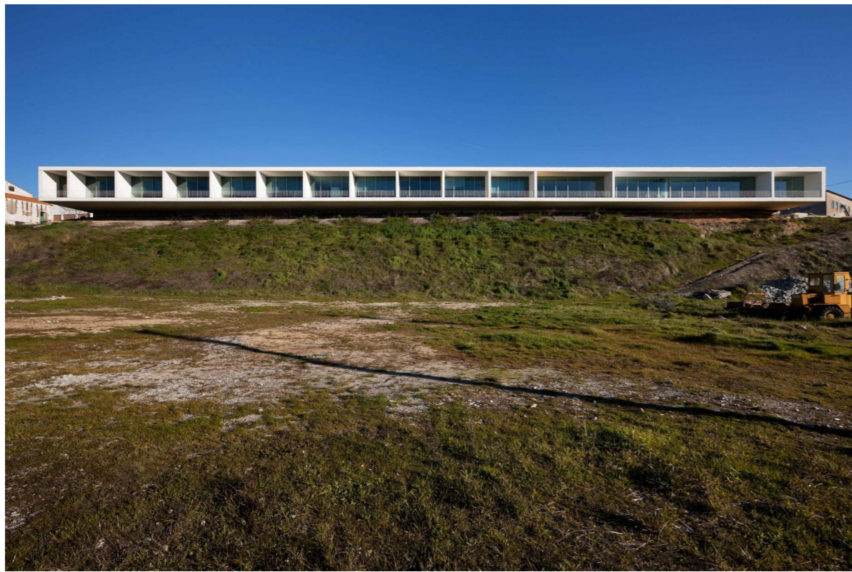
Catering School and Auditorium - Portalegre, Portugal
