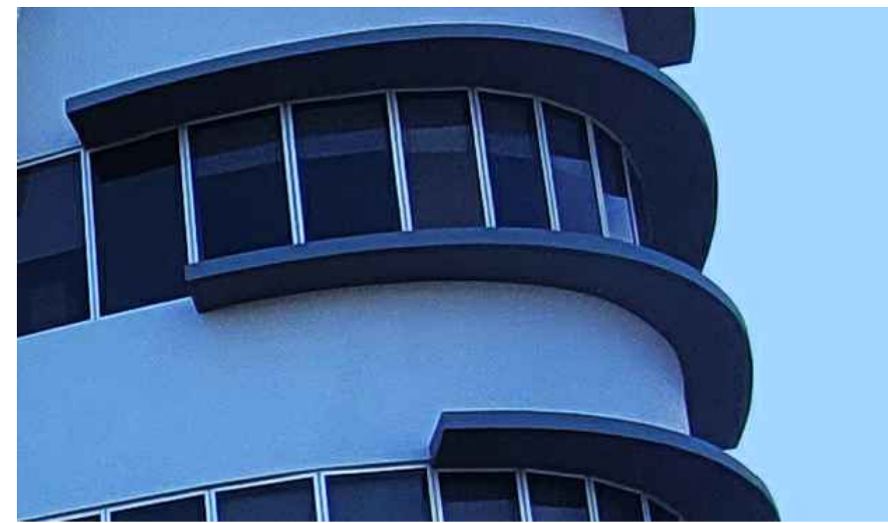
② EXISTING OFFICE BUILDING EYEBROW
