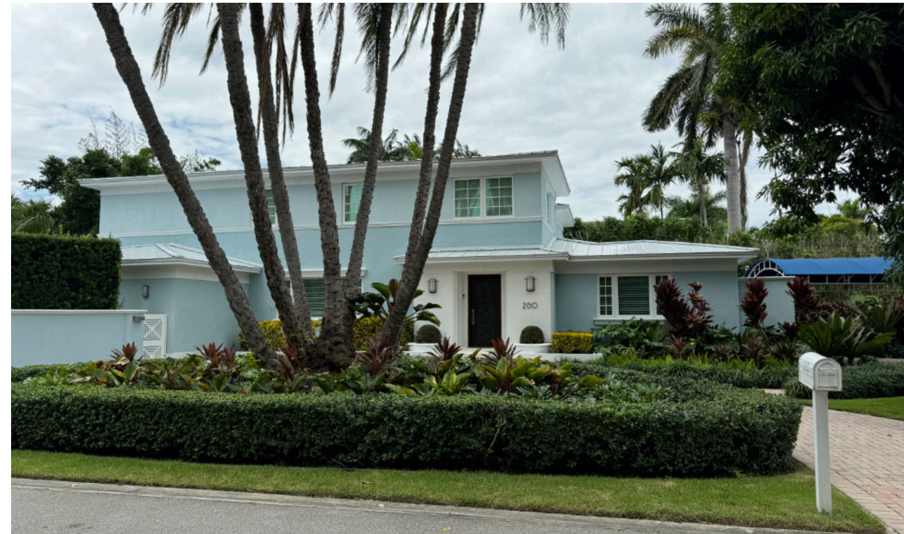
4 2130 REGATTA AVENUE EXISTING TWO-STORY RESIDENCE
