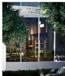
2 ALUMINUM-FRAMED STOREFRONT SYSTEM, W/ IMPCT-RESISTANT GLASS
