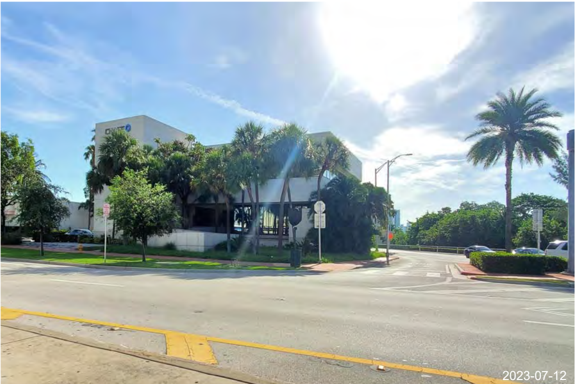
14. VIEW OF CHASE BANK SOUTH OF SITE
