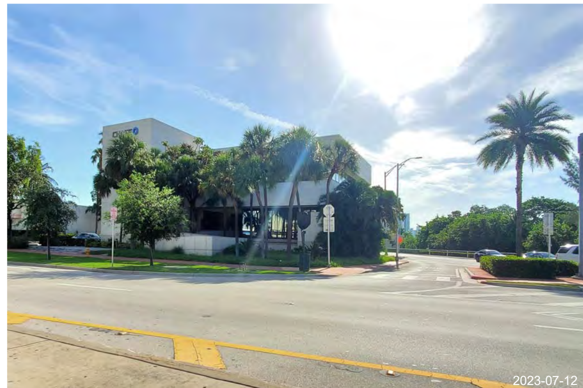
14. VIEW OF CHASE BANK SOUTH OF SITE
