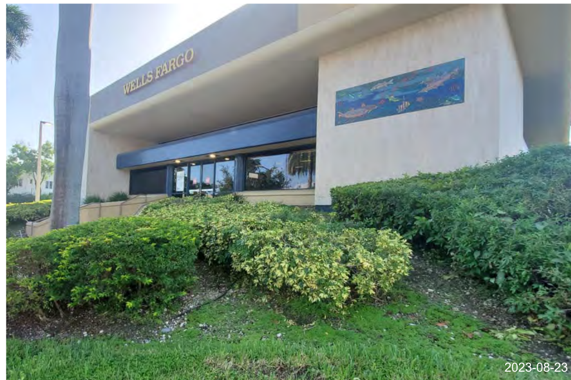
17. WELLS FARGO ENTRANCE ON ALTON RD.
