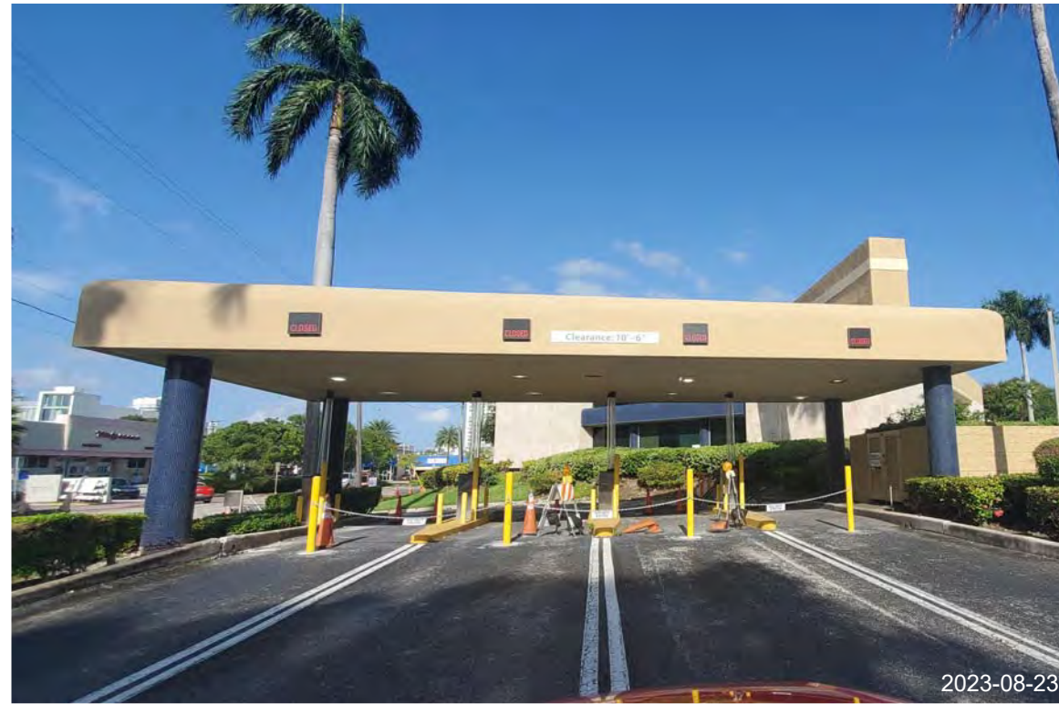
23. EXISTING DRIVE THRU BANK ON SITE
