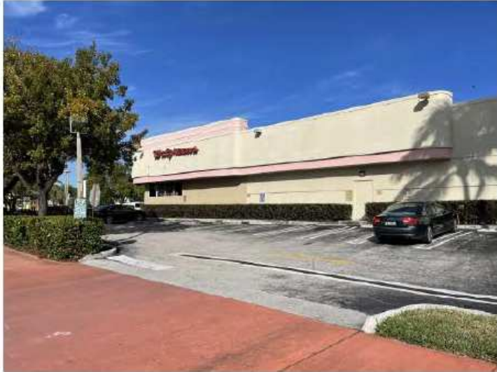
22 ALTON ROAD LOOKING NORTH EAST AT WALGREENS
