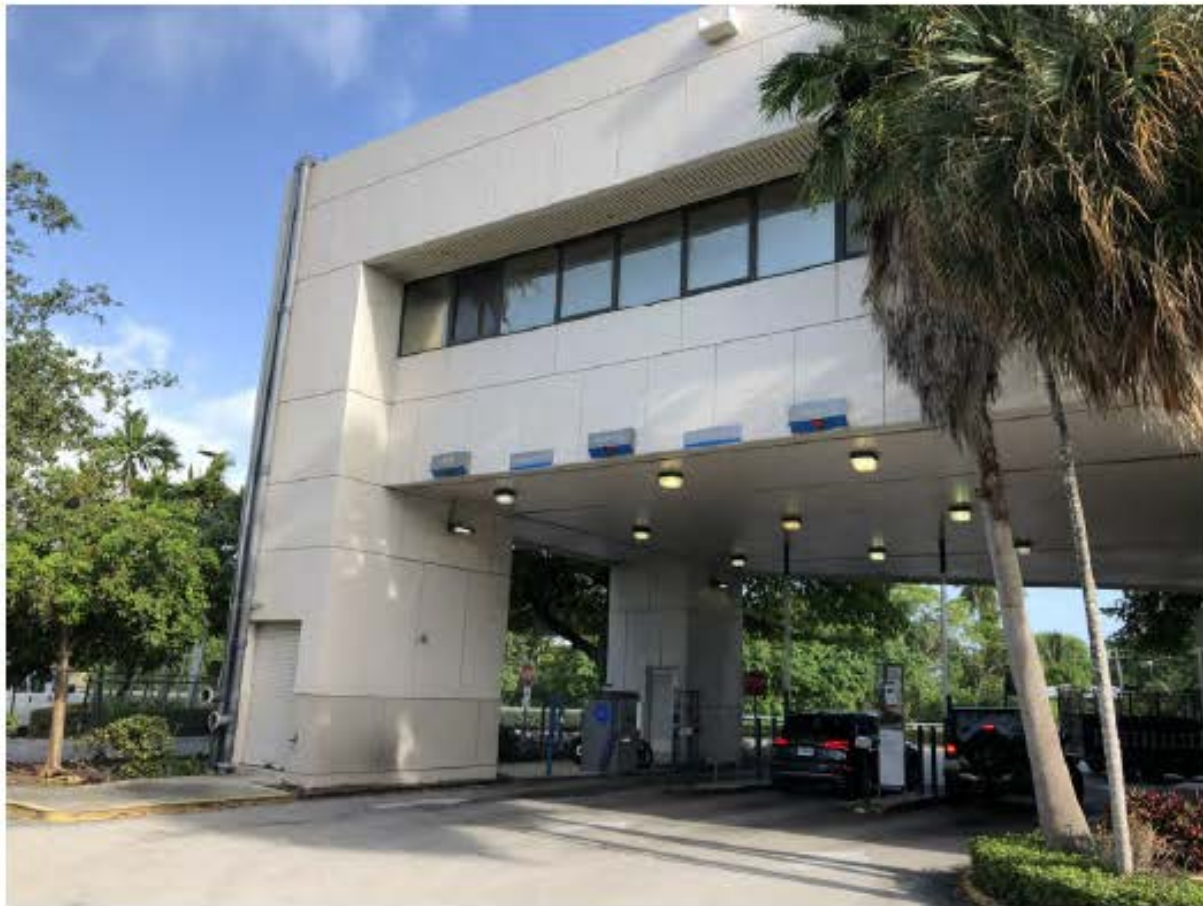
11 EXISTING PARKING LOOKING SOUTHEAST
