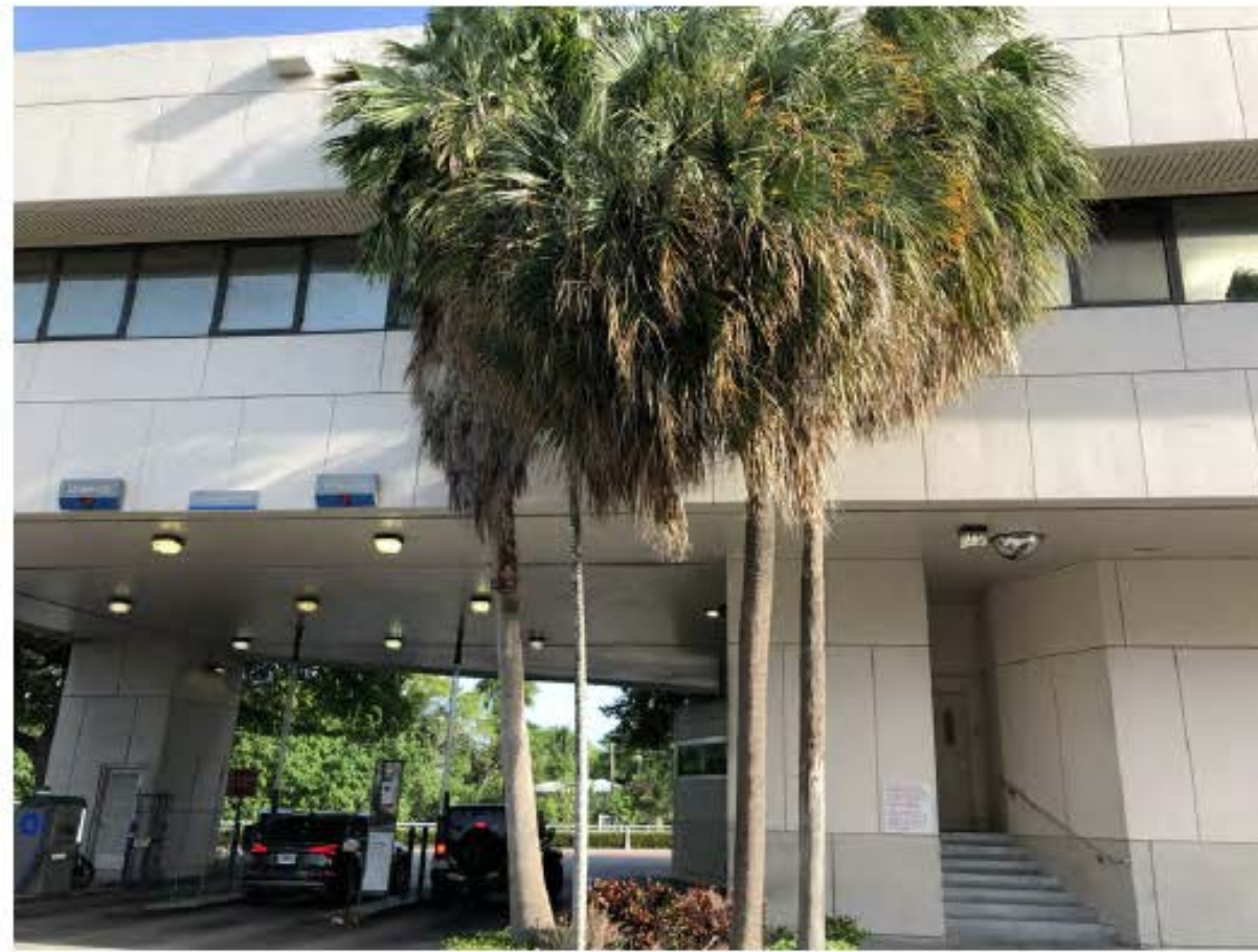
10 EXISTING PARKING LOOKING SOUTH
