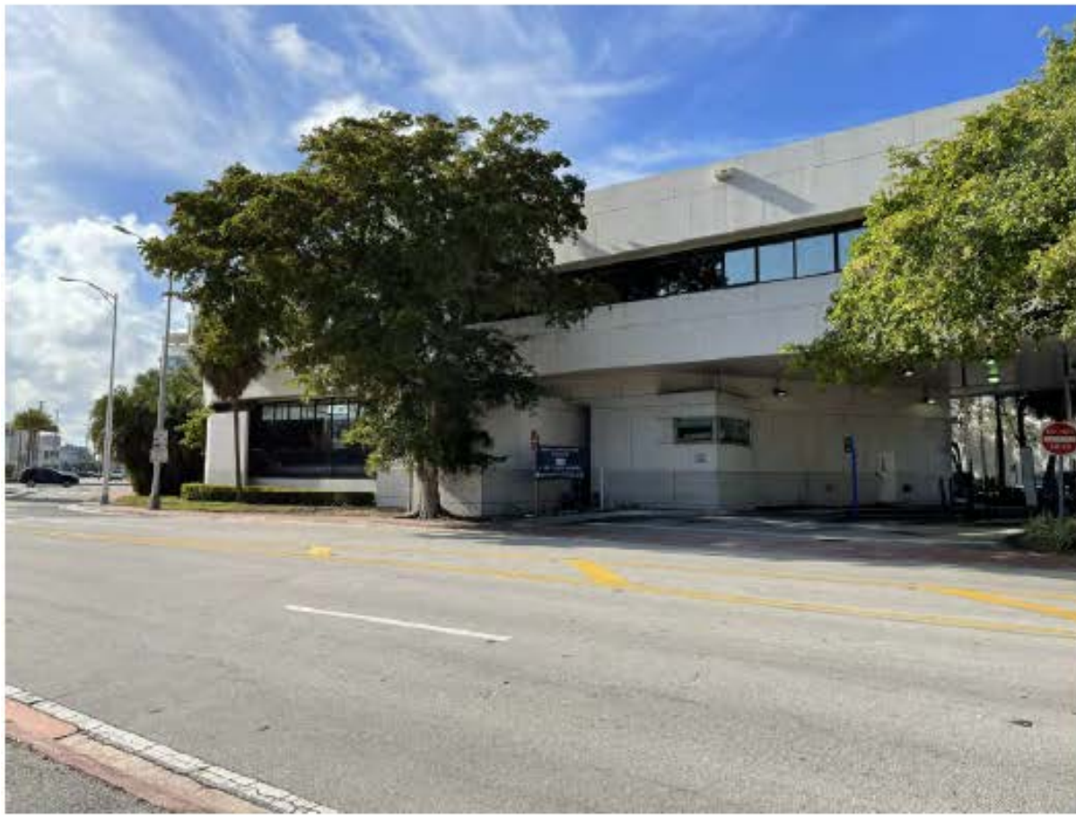
05 DADE BOULEVARD LOOKING NORTHWEST
