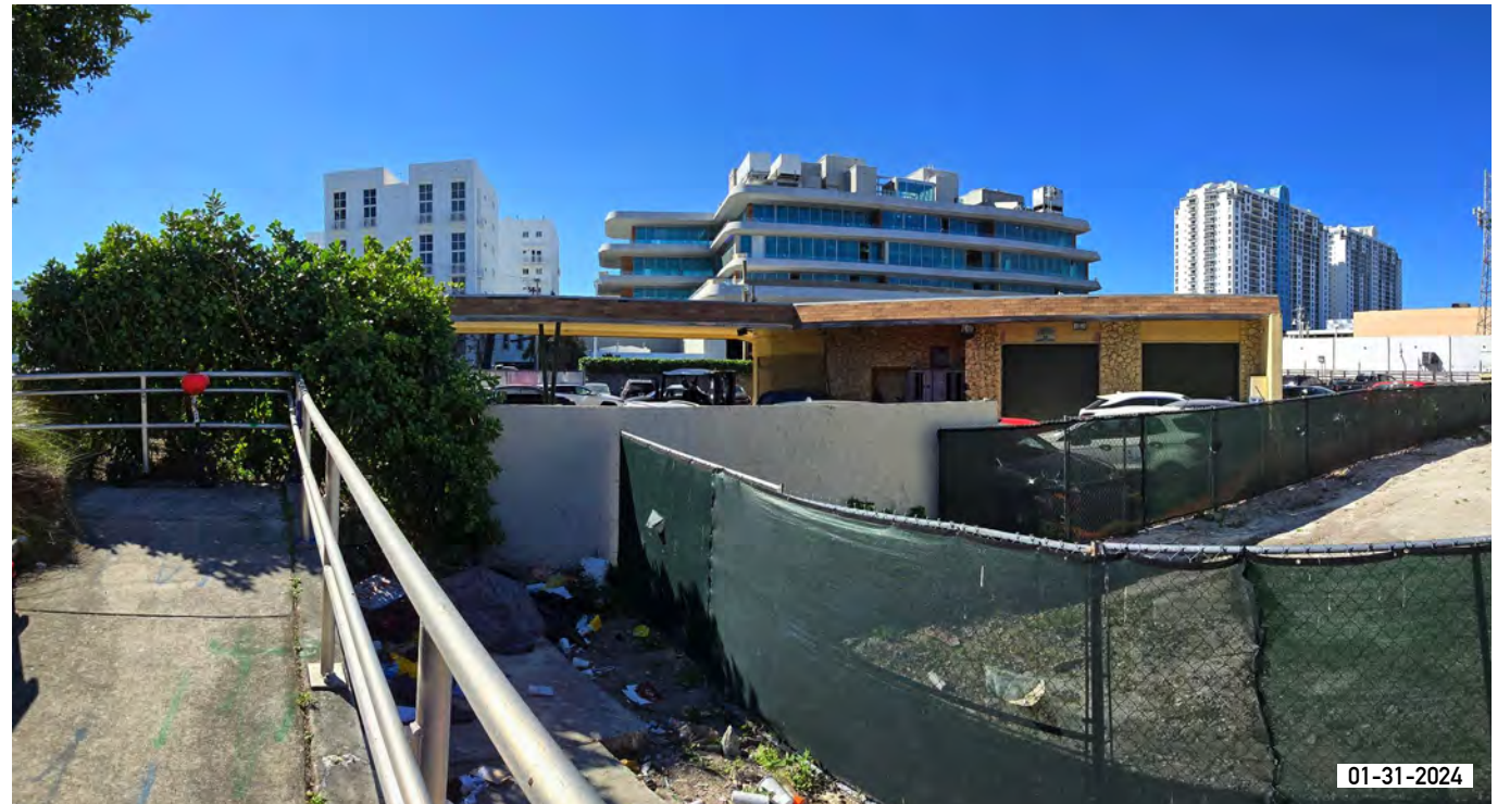
15. SOUTH ENTRANCE AND RAMP
