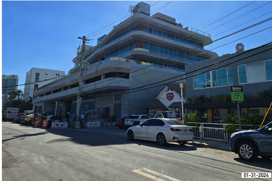
7. VIEW TOWARDS CONSTRUCTION SITE
