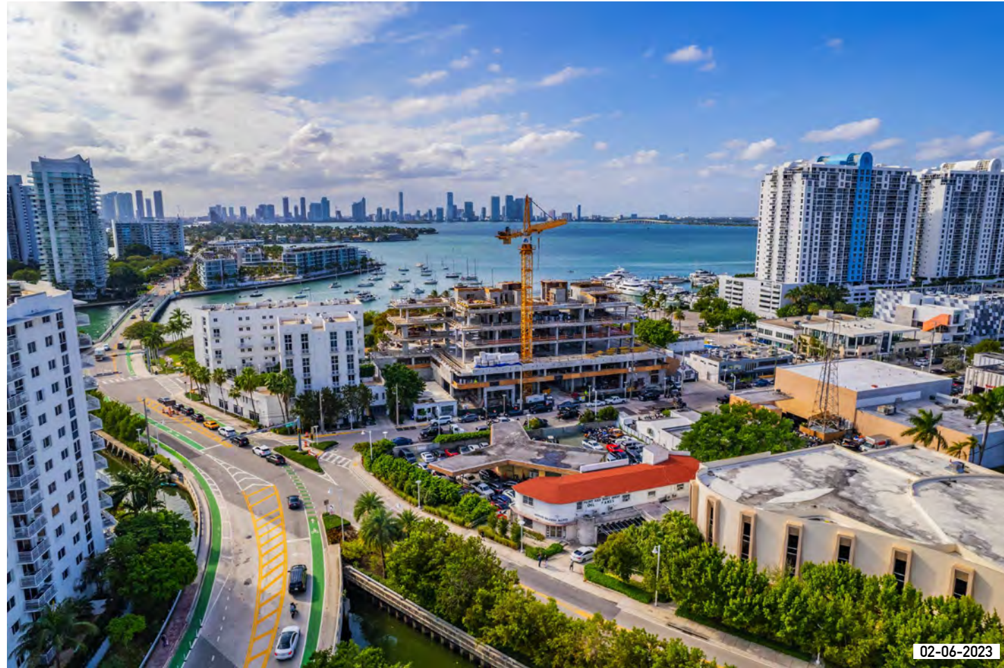
1. SITE AERIAL PHOTO BEFORE DEMOLITION
