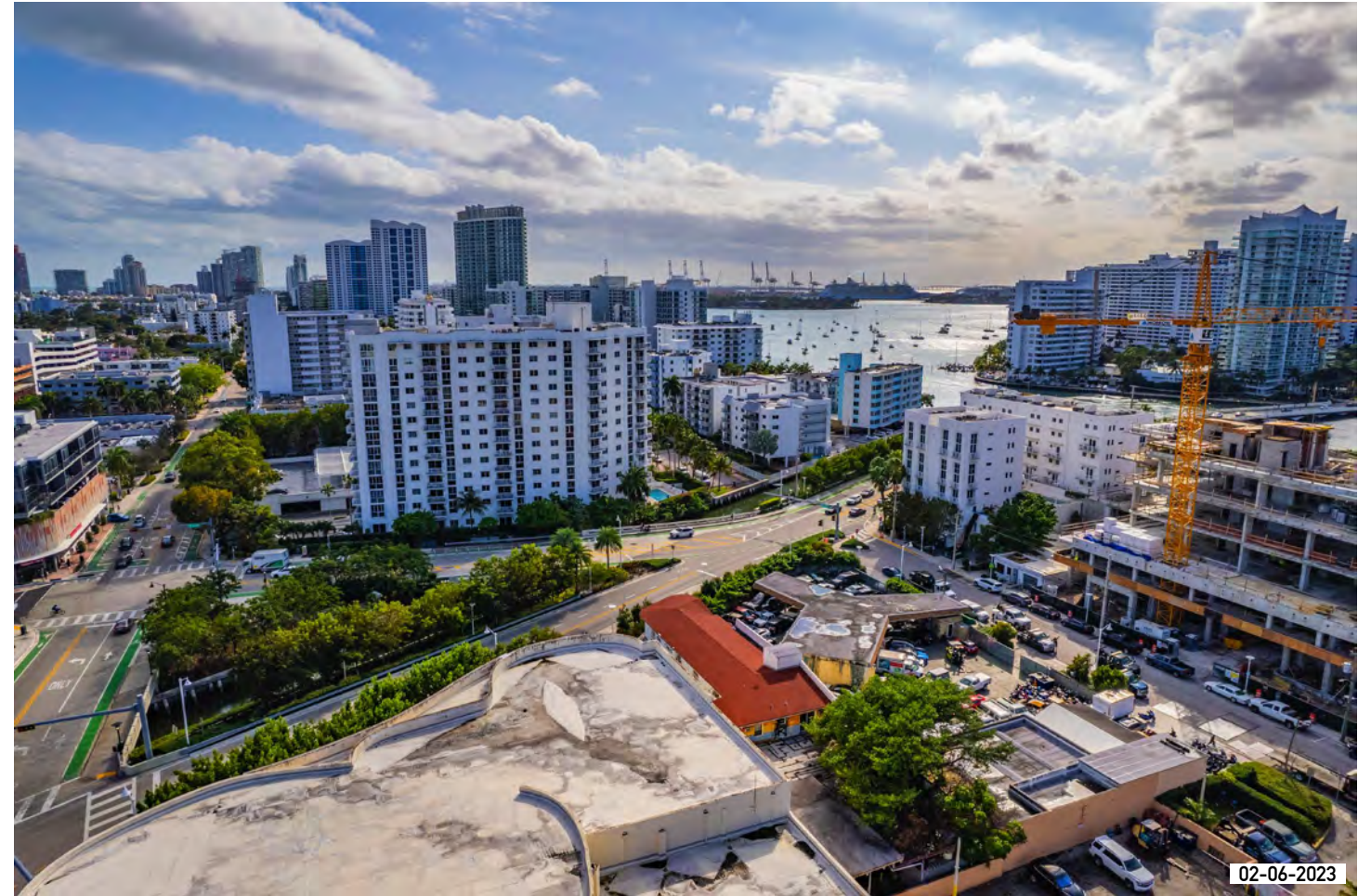
2. SITE AERIAL PHOTO BEFORE DEMOLITION
