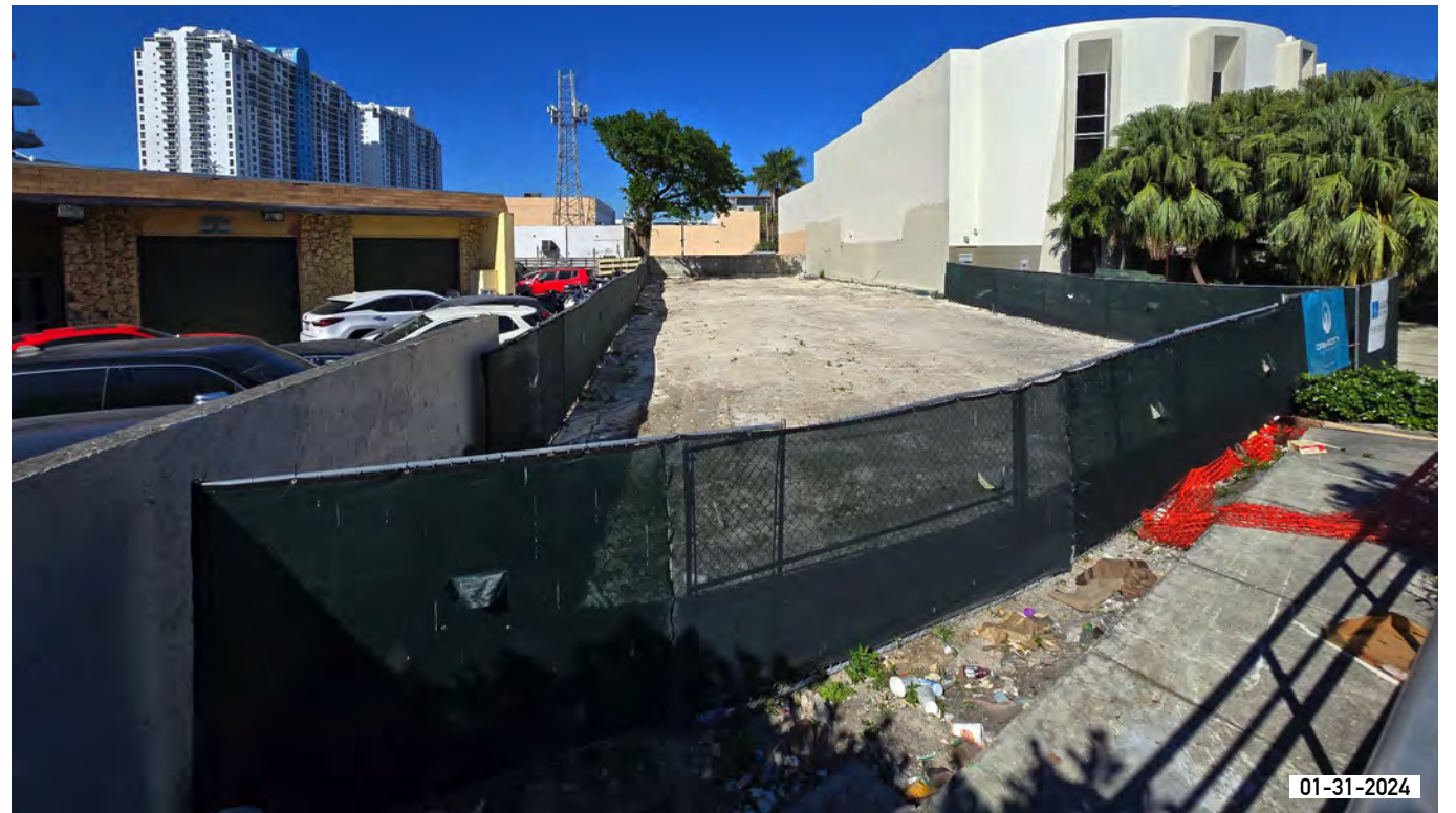
17. FRONT VIEW FROM DADE BOULEVARD
