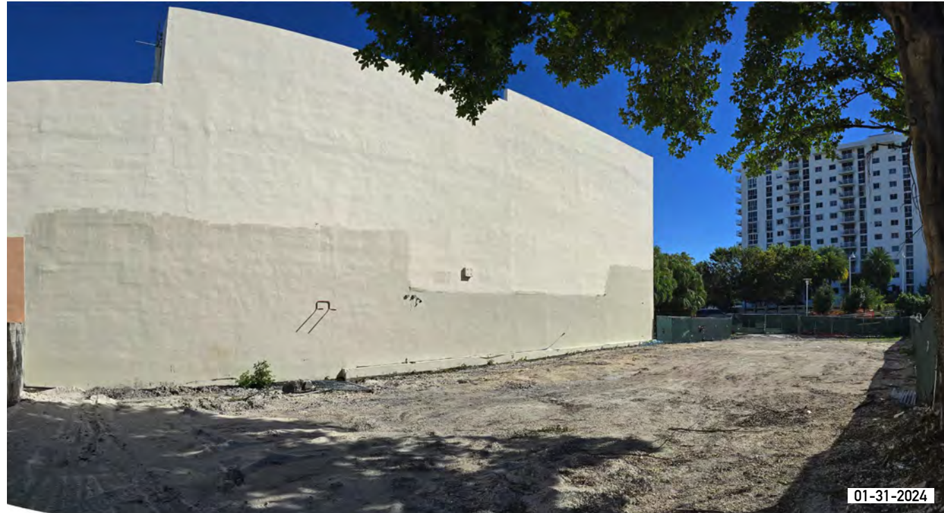
14. SOUTH WEST CORNER OF SITE
