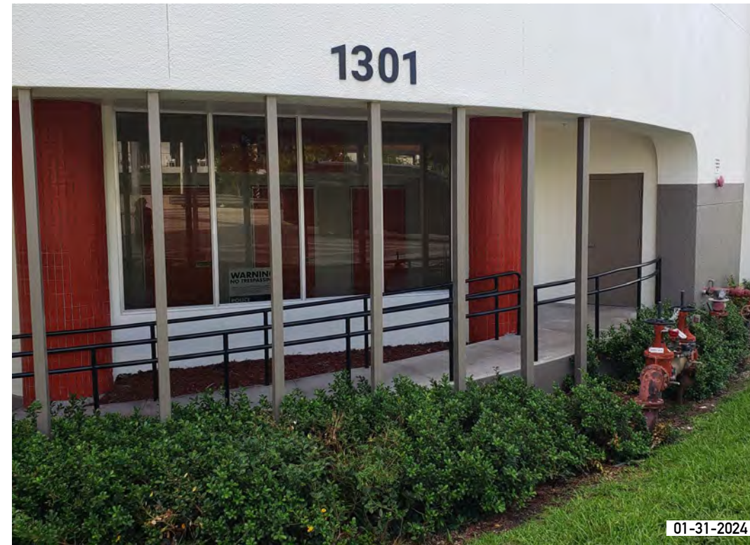
21. CORNER ENTRANCE FROM DADE BOULEVARD AND WEST AVENUE
