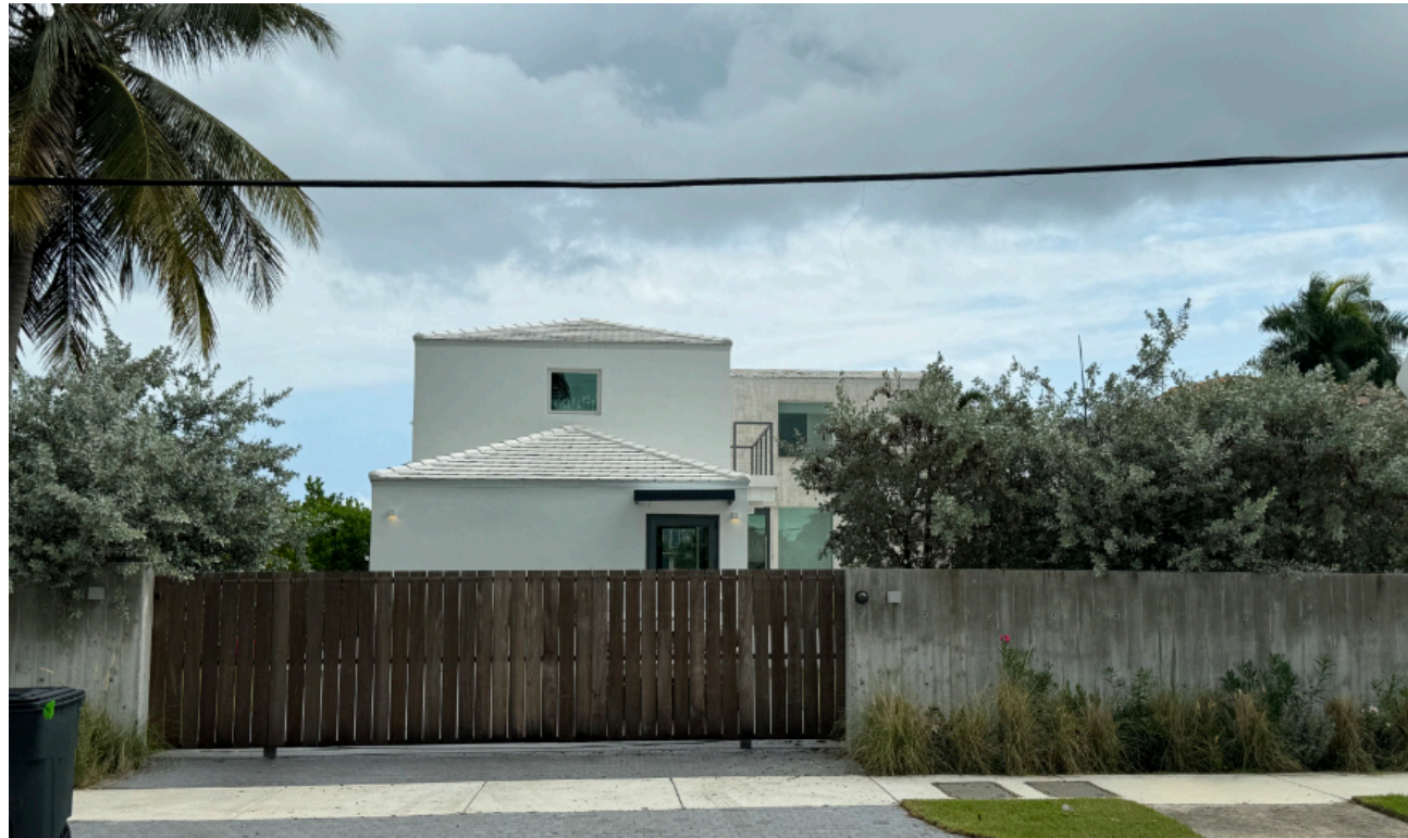
5 403 E. DI LIDO DRIVE EXISTING TWO-STORY RESIDENCE
