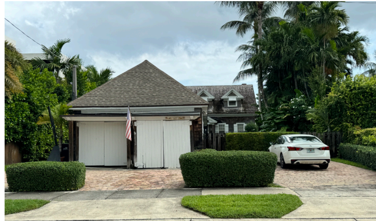
8 315 E. DI LIDO DRIVE EXISTING TWO-STORY RESIDENCE
