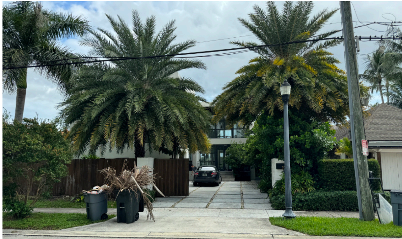
7 321 E. DI LIDO DRIVE EXISTING TWO-STORY RESIDENCE
