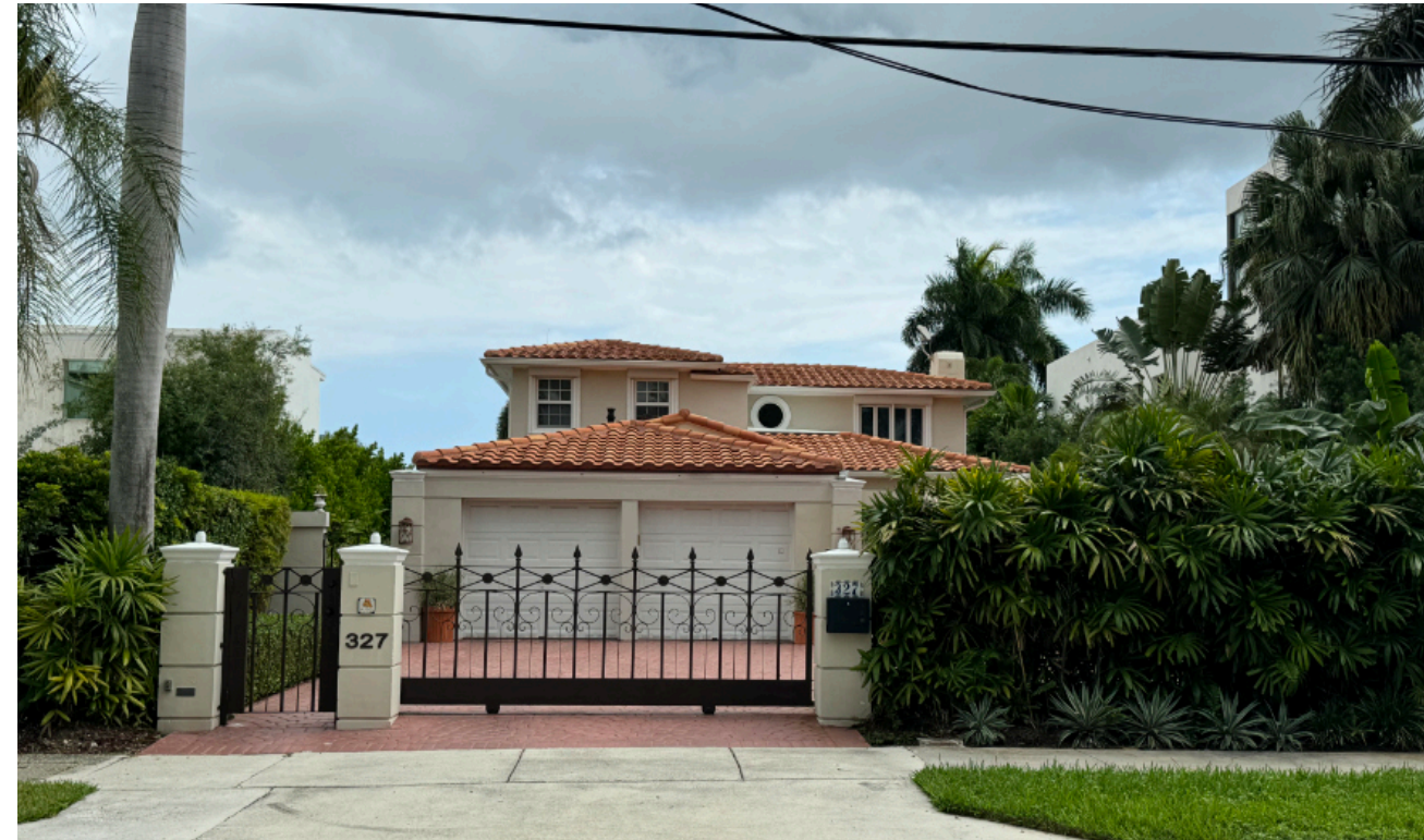
6 327 E. DI LIDO DRIVE EXISTING TWO-STORY RESIDENCE
