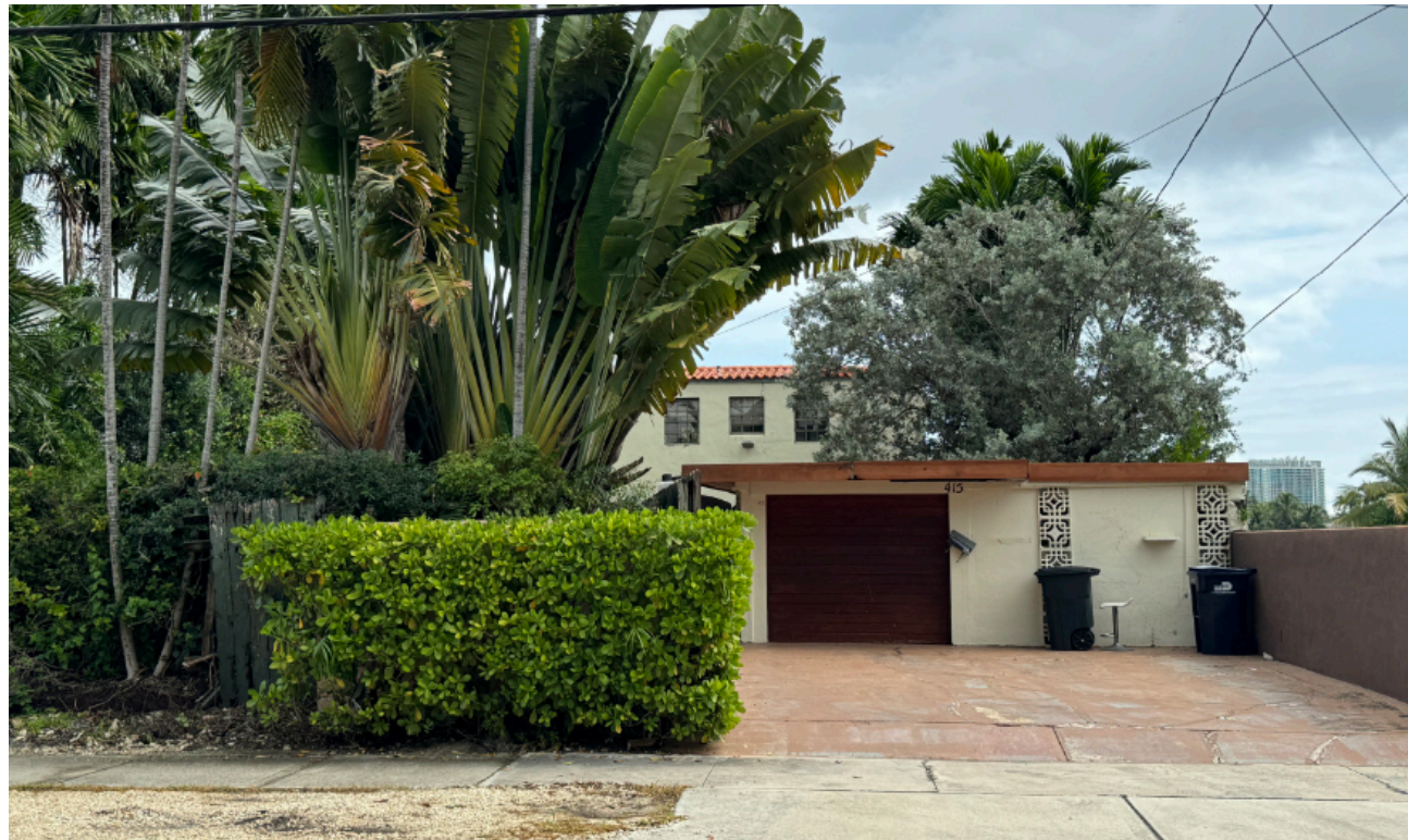
3 415 E. DI LIDO DRIVE EXISTING TWO-STORY RESIDENCE
