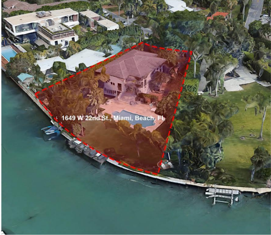
REAR AERIAL VIEW
