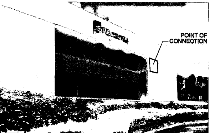
7 EXISTING SOUTH VIEW
