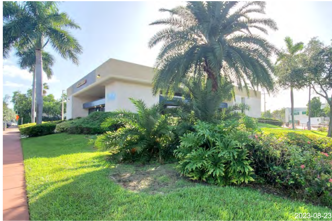
19. VIEW OF SITE FROM ALTON RD. AND 19TH ST INTERSECTION
