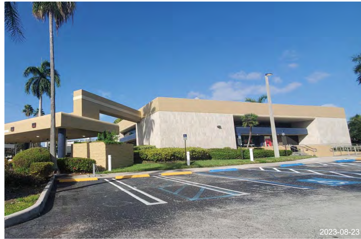
24. VIEW OF WELLS FARGO FROM EXISTING PARKING
