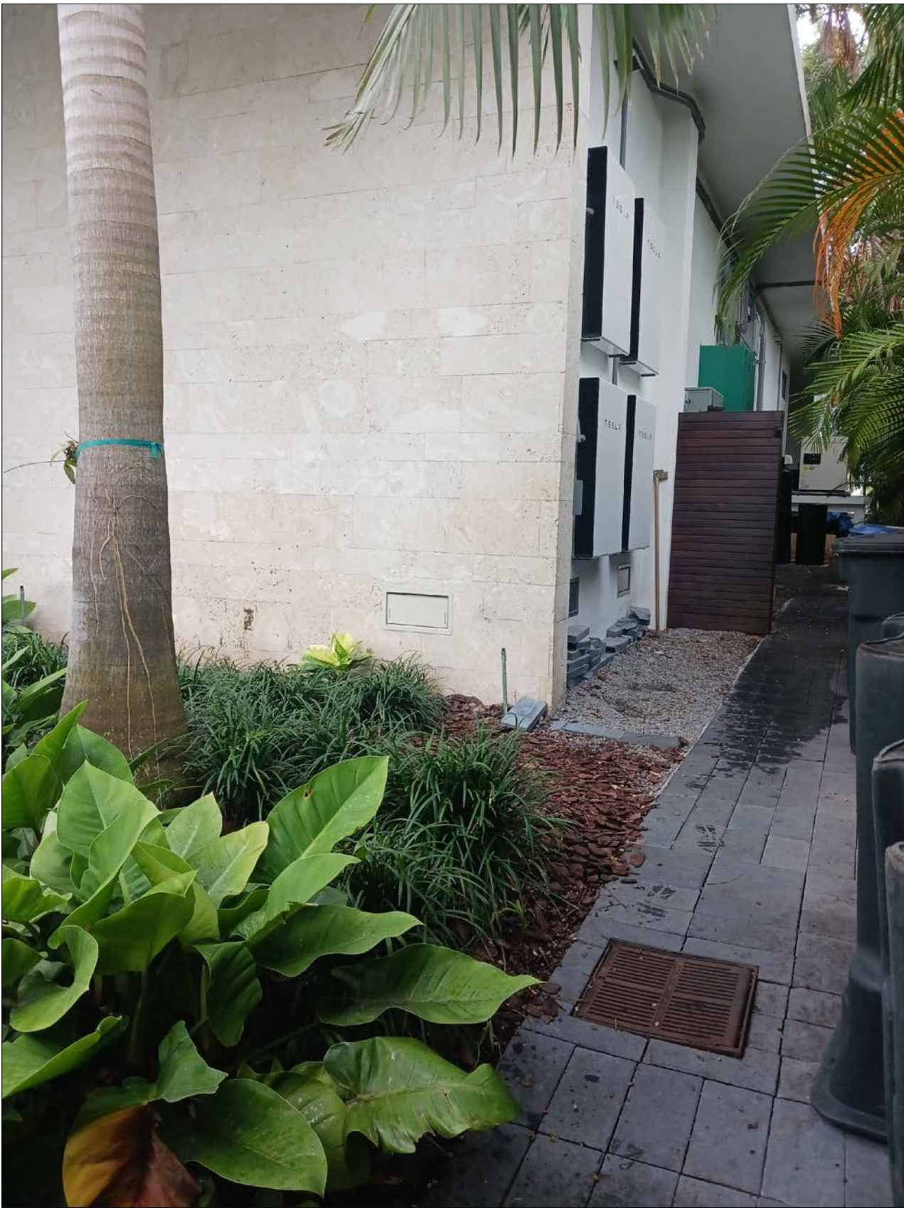
② SIDE LOOKING SOUTHEAST
