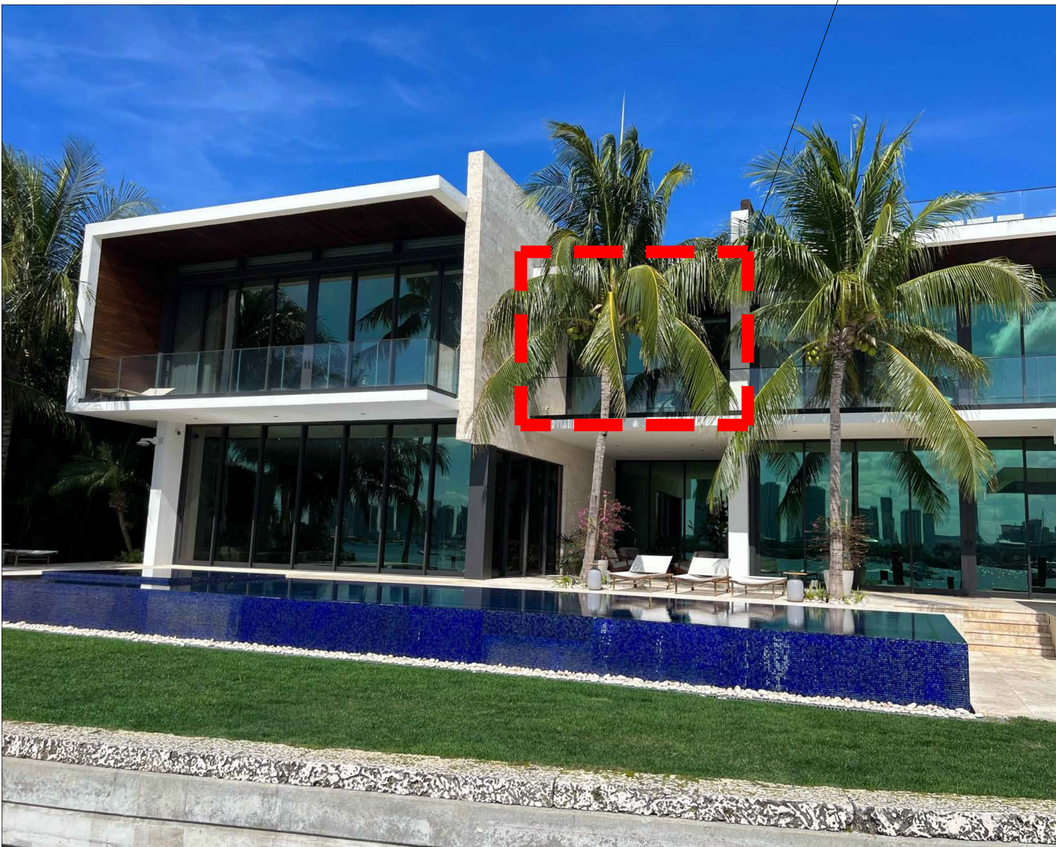
① REAR - LOOKING NORTH EXISTING
