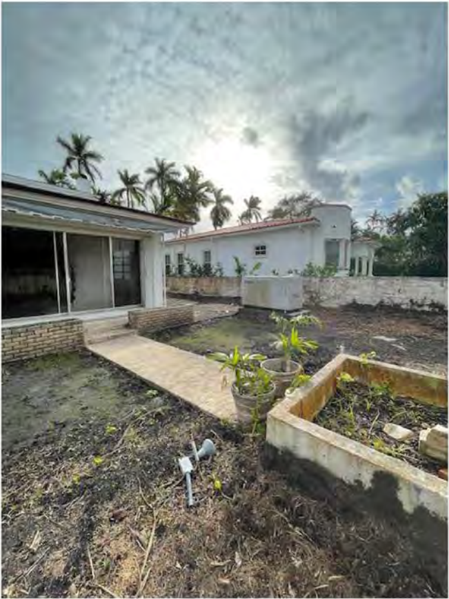
REAR FACING SOUTH
