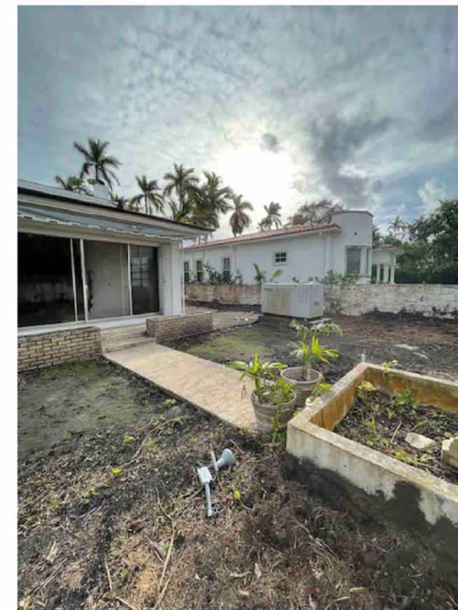
REAR FACING SOUTH
