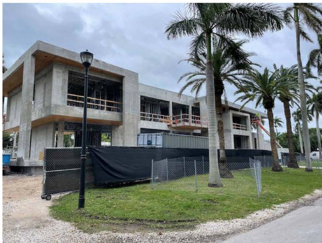
MODERN HOUSE ON LA GORCE ISLAND UNDER CONSTRUCTION
