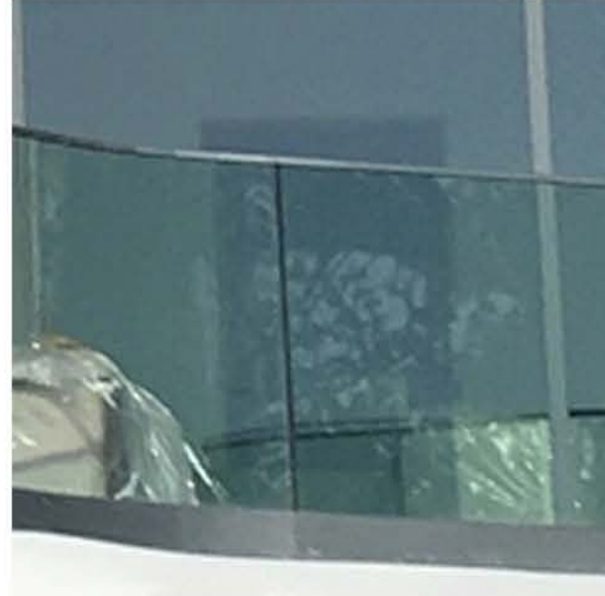
GLR IMPACT GLASS HANDRAIL- CLEAR, RADIUS CORNERS
