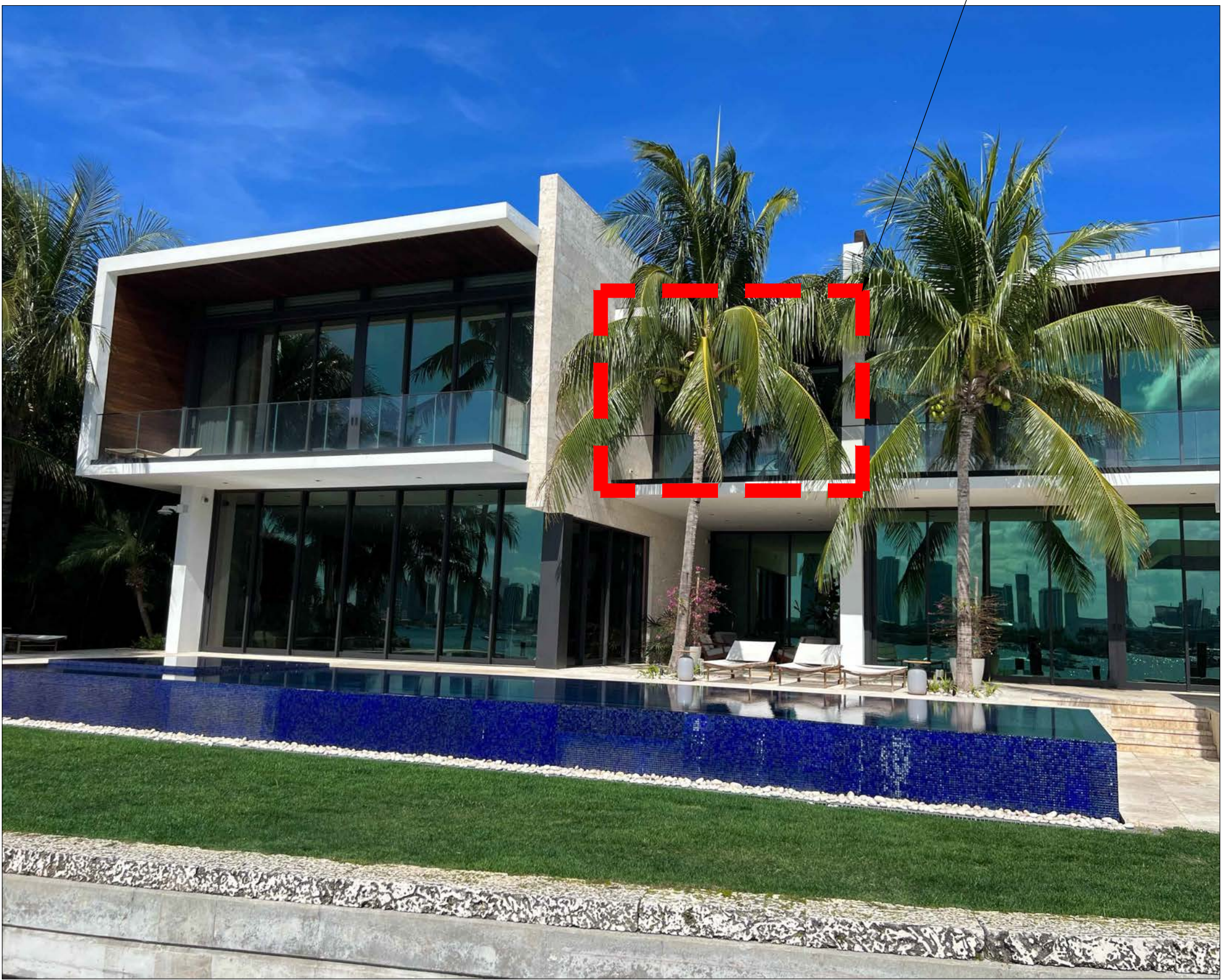
① REAR - LOOKING NORTH EXISTING
