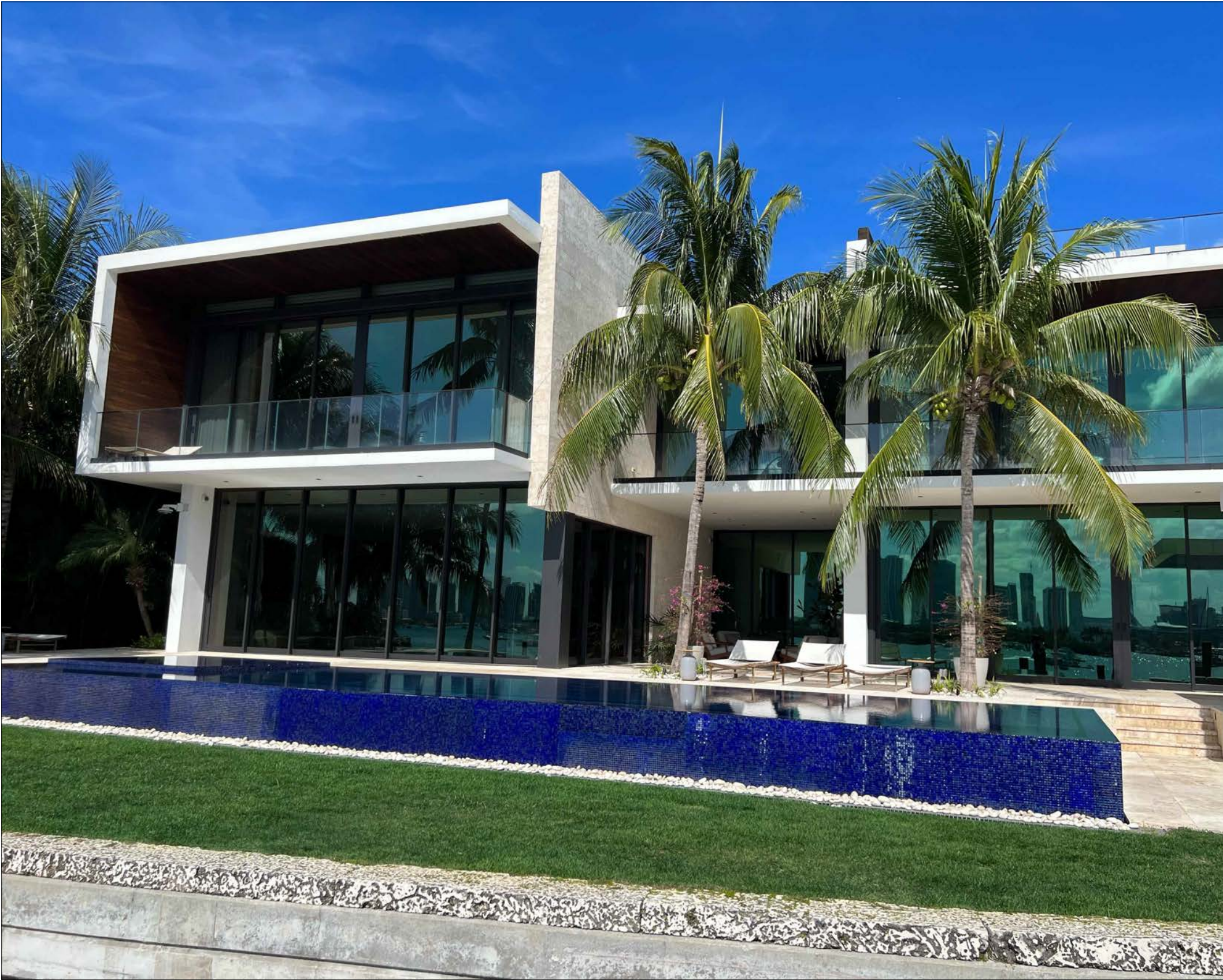
④ REAR - LOOKING NORTH
