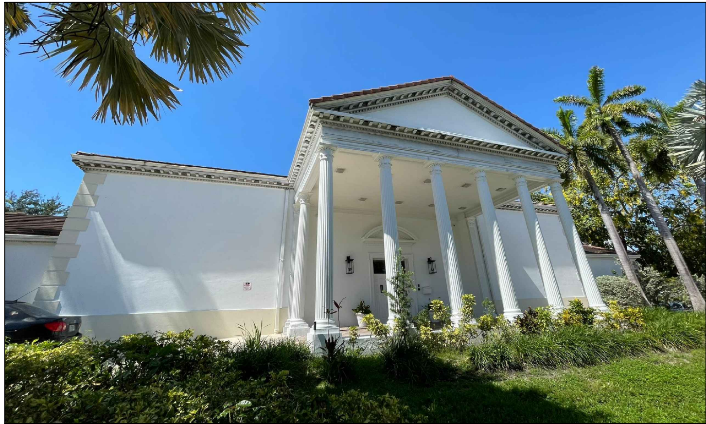
NORTH (FRONT VIEW)
