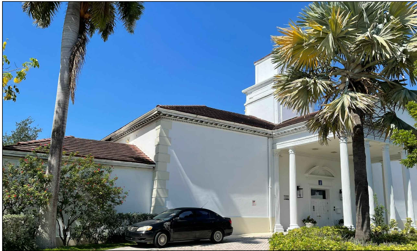
NORTHEAST (FRONT VIEW)
