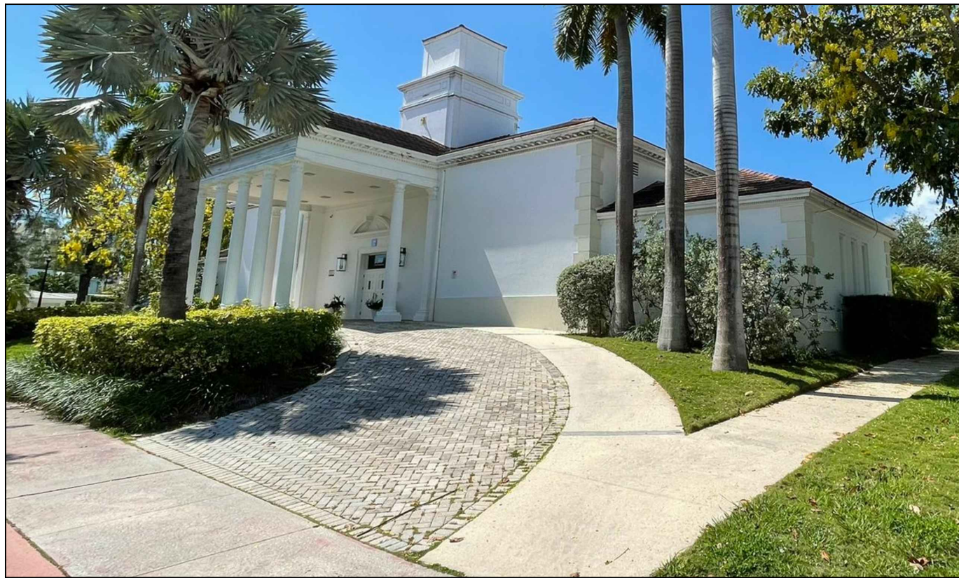
NORTHWEST (FRONT VIEW)
