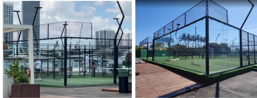
PADEL COURT FENCE AND COURT FELT
