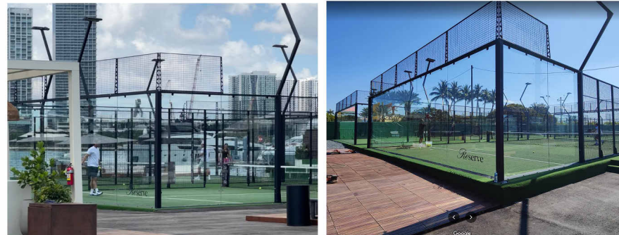
PADEL COURT FENCE AND COURT FELT
