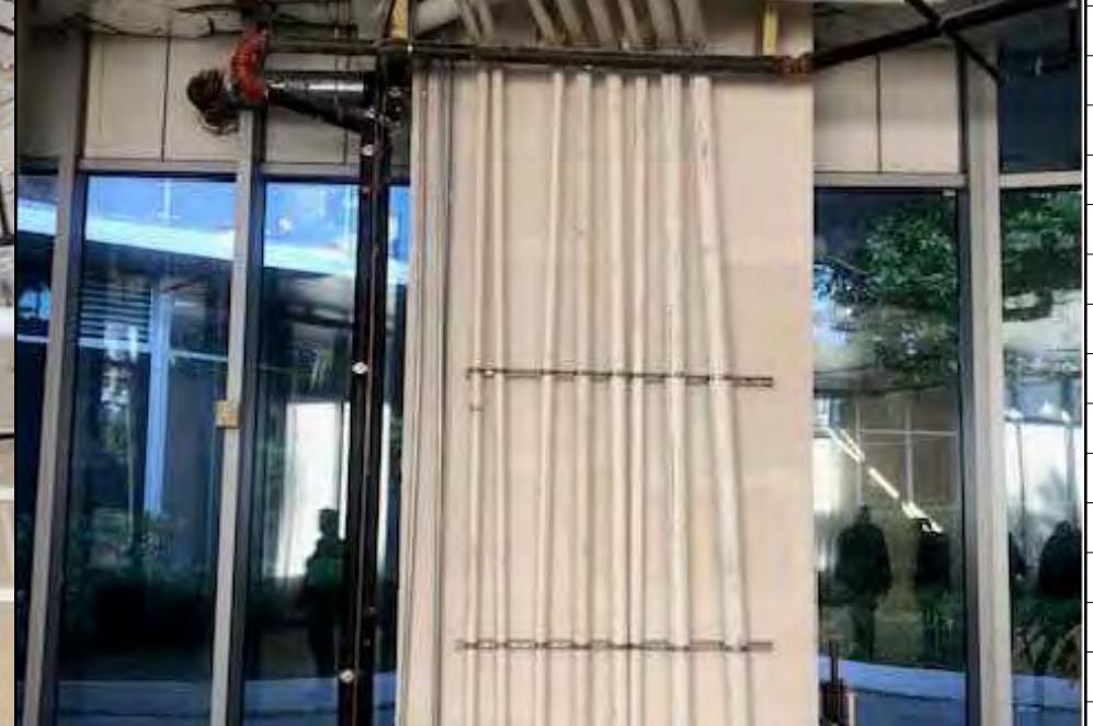
H INTERIOR - EXISTING CONDITIONS SCALE: NTS
