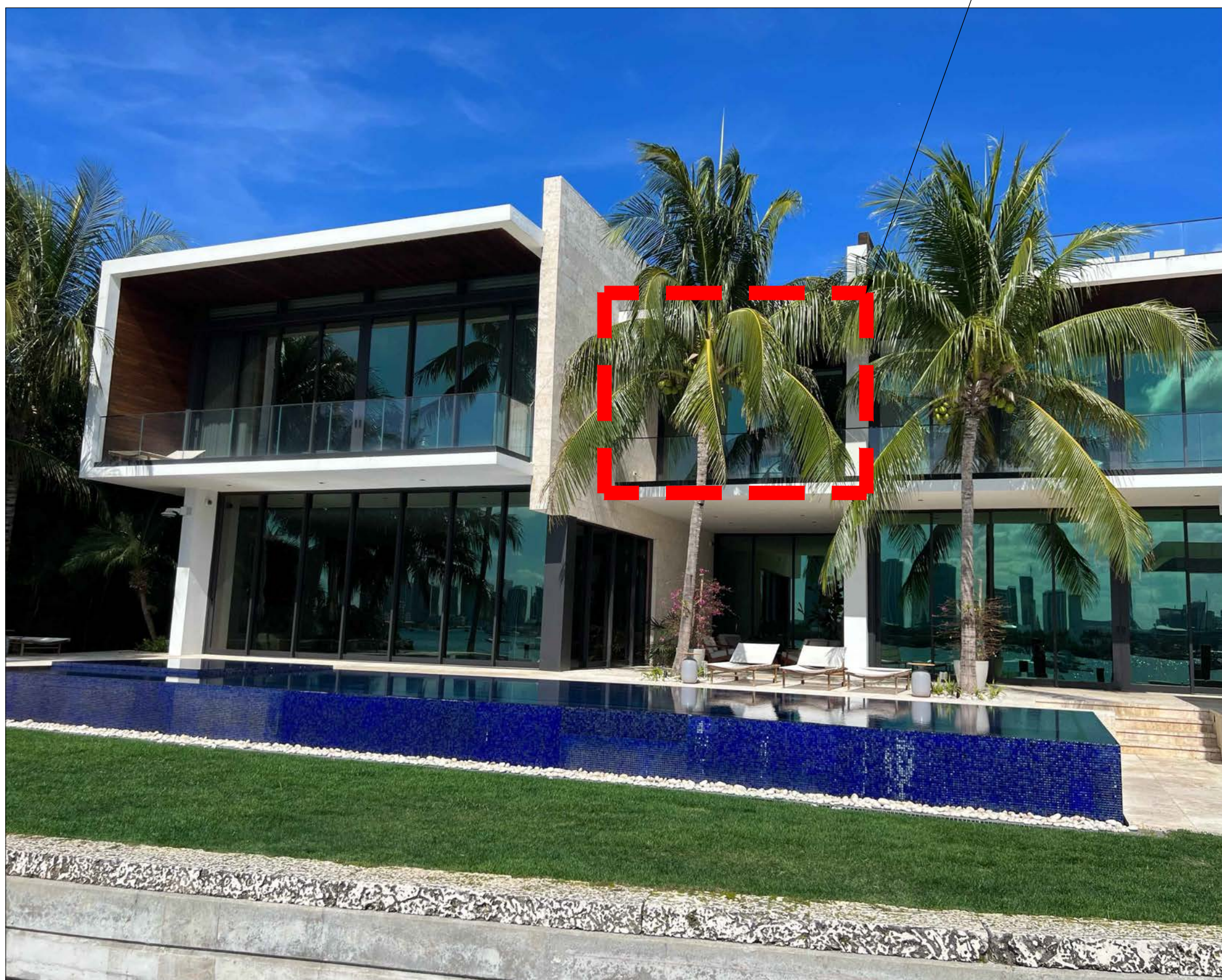
① REAR - LOOKING NORTH EXISTING
