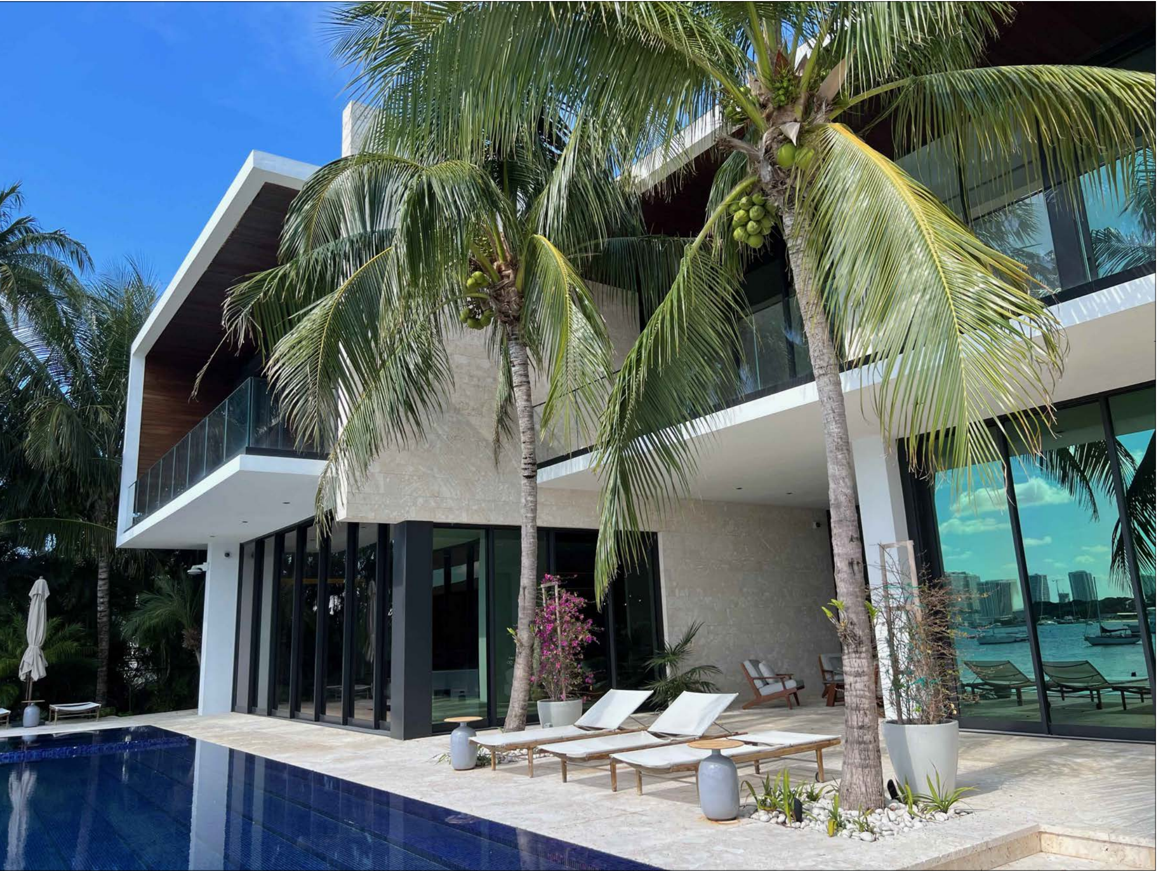
④ REAR - LOOKING NORTHWEST
