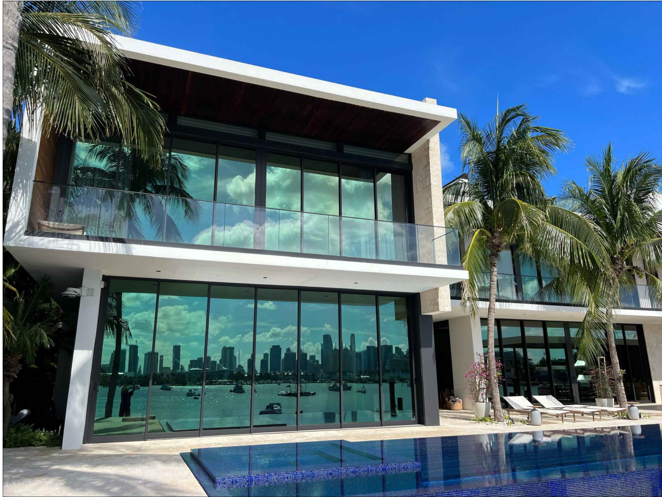
③ REAR LOOKING NORTH
