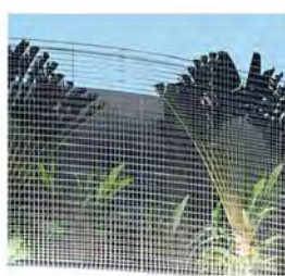
3 S.S. OR ALUMINUM SQUARE PENING WIRE MESH PAINTED WHITE. OPENINGS 4"
