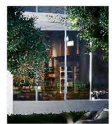
2 ALUMINUM-FRAMED STOREFRONT SYSTEM, W/ IMPCT-RESISTANT GLASS
