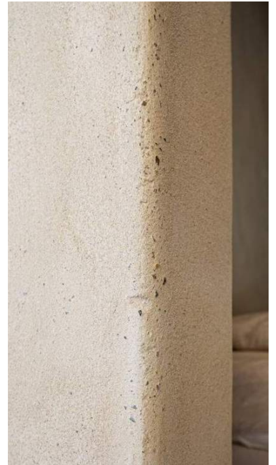
WALLS AND SOFFITS - ACRYLIC PLASTER
