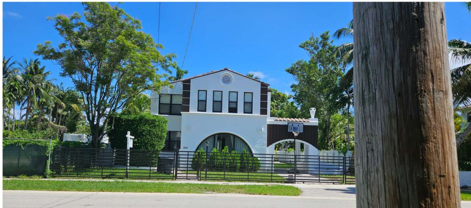
3035 NORTH BAY ROAD
