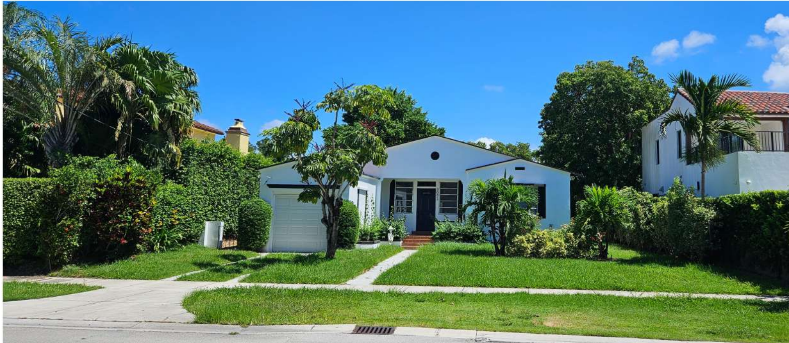
3093 NORTH BAY ROAD
