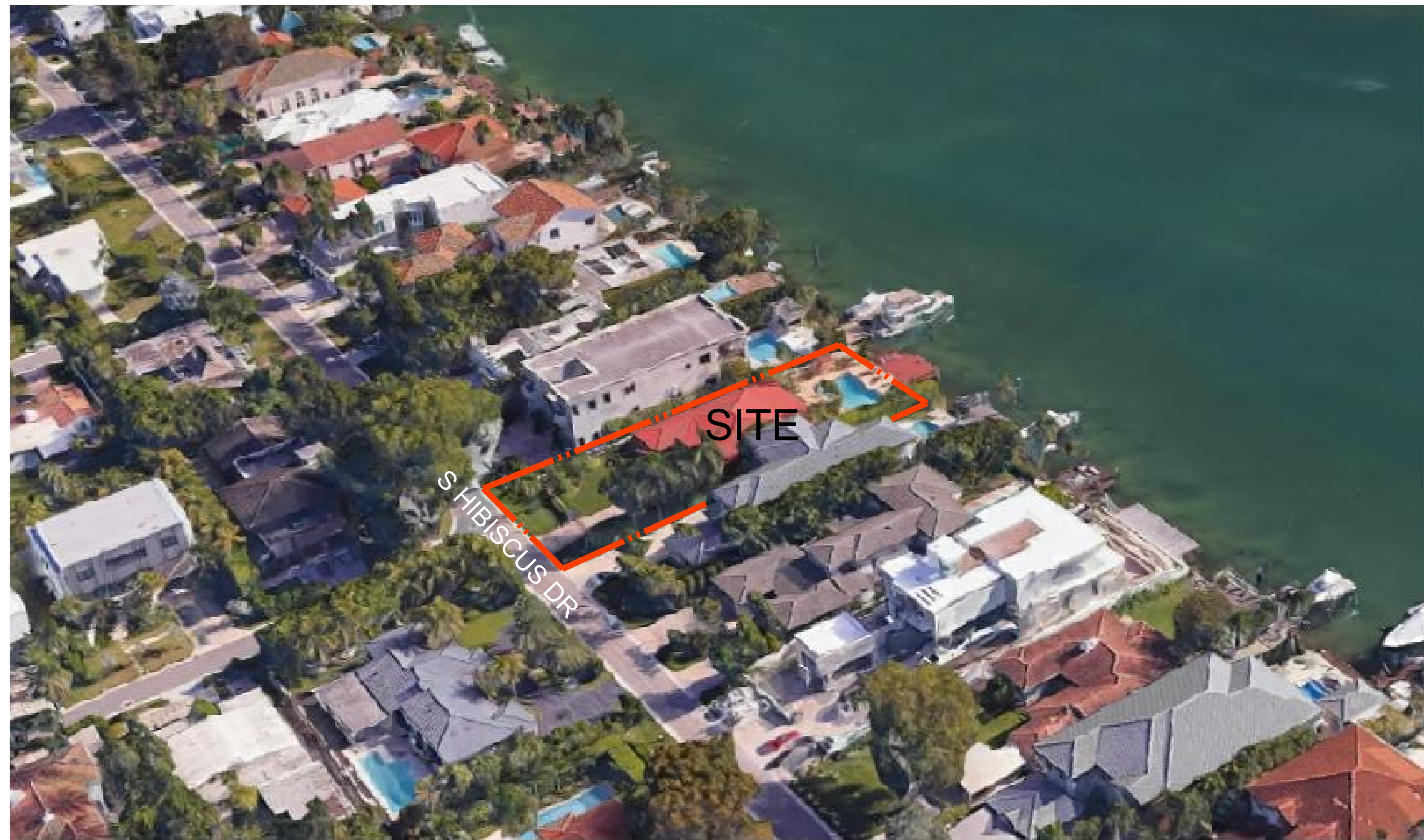
FRONT AERIAL (NW) VIEW
