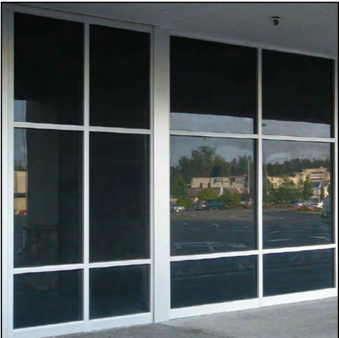
1 APPLIED OPAQUE BLACK FILM ON STOREFRONT GLAZING ELEVATION FACING THE CONDO GARDEN
