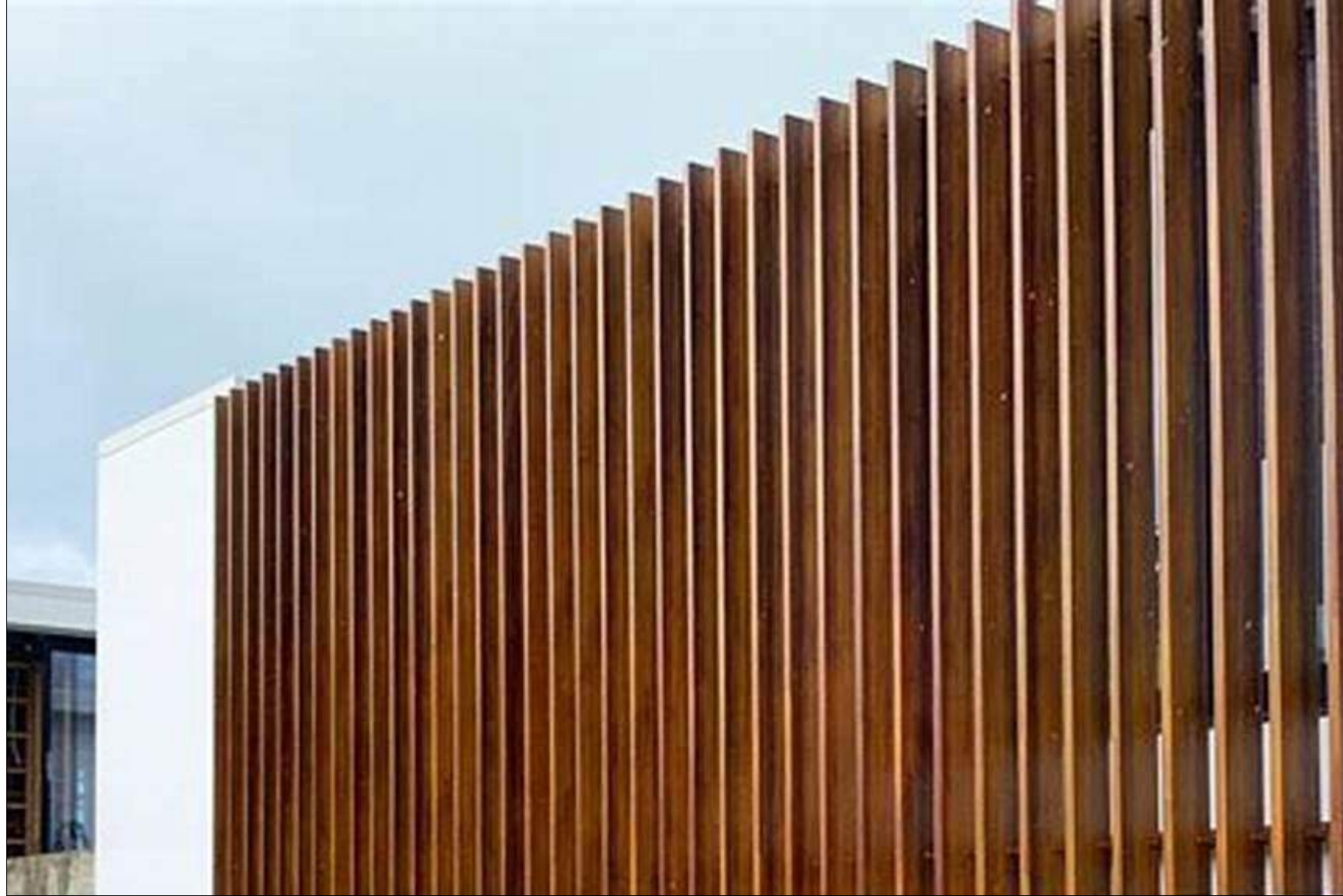
ALUMINUM GARAGE CLADDING AND BRISE SOLEIL
