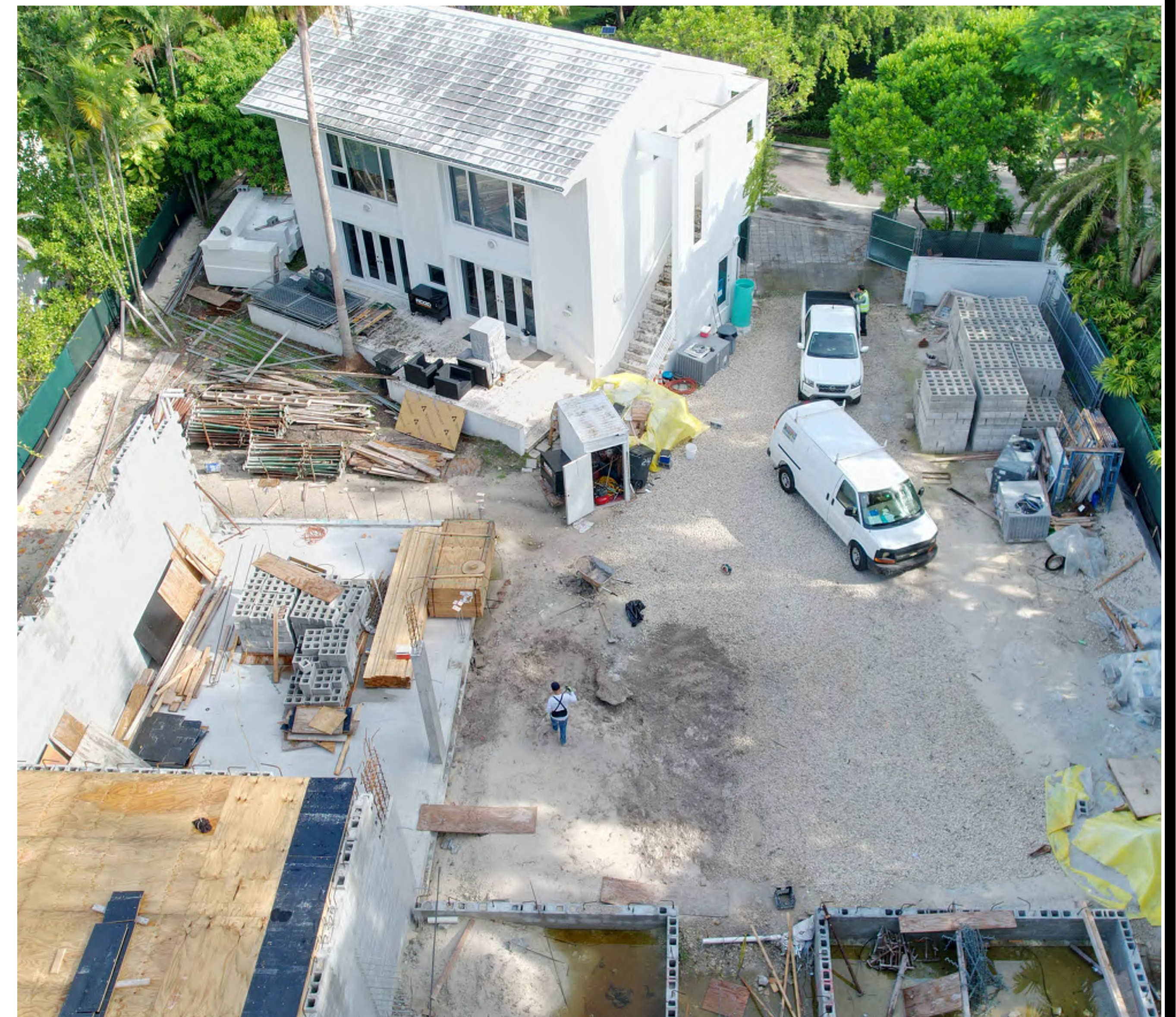
03 GUEST HOUSE - AERIAL SITE PHOTO (10/10/2023)
