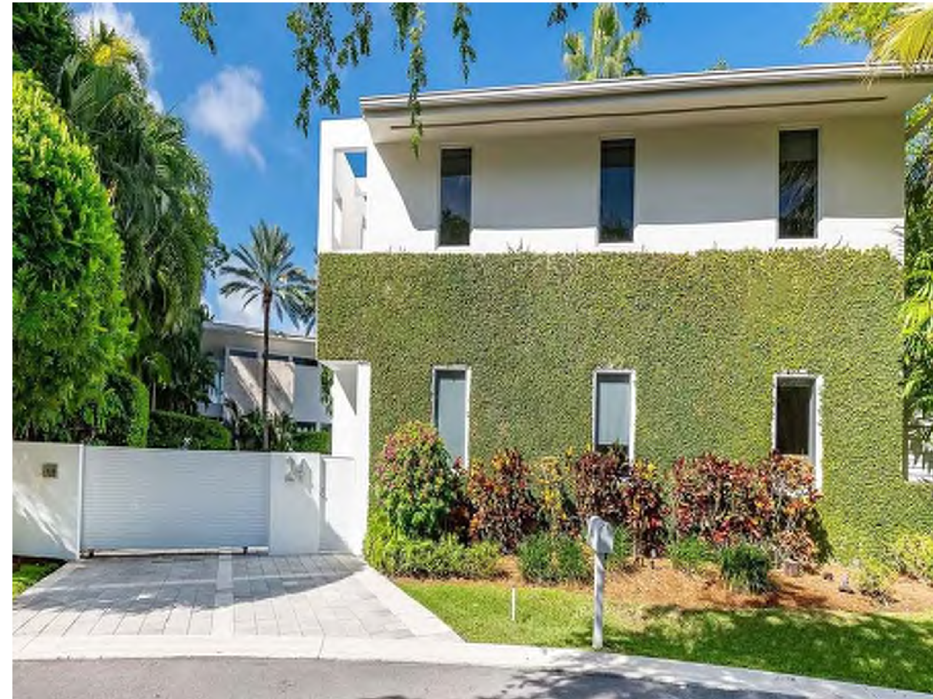
07 24 PALM AVENUE (5/23/2022) PRIOR TO CONSTRUCTION
