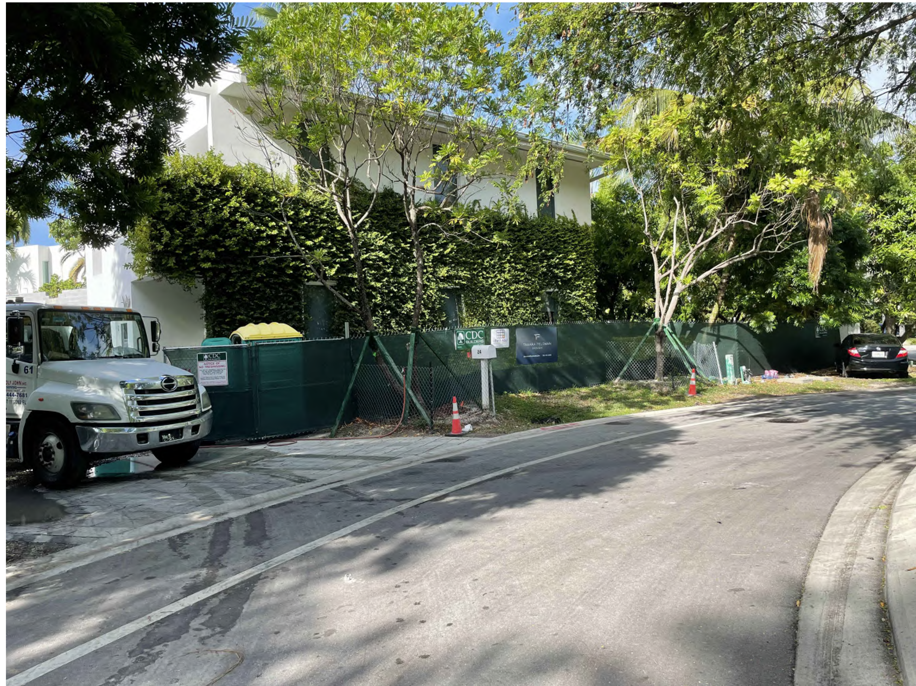
07 24 PALM AVENUE (11/3/2023) CURRENTLY UNDER CONSTRUCTION
