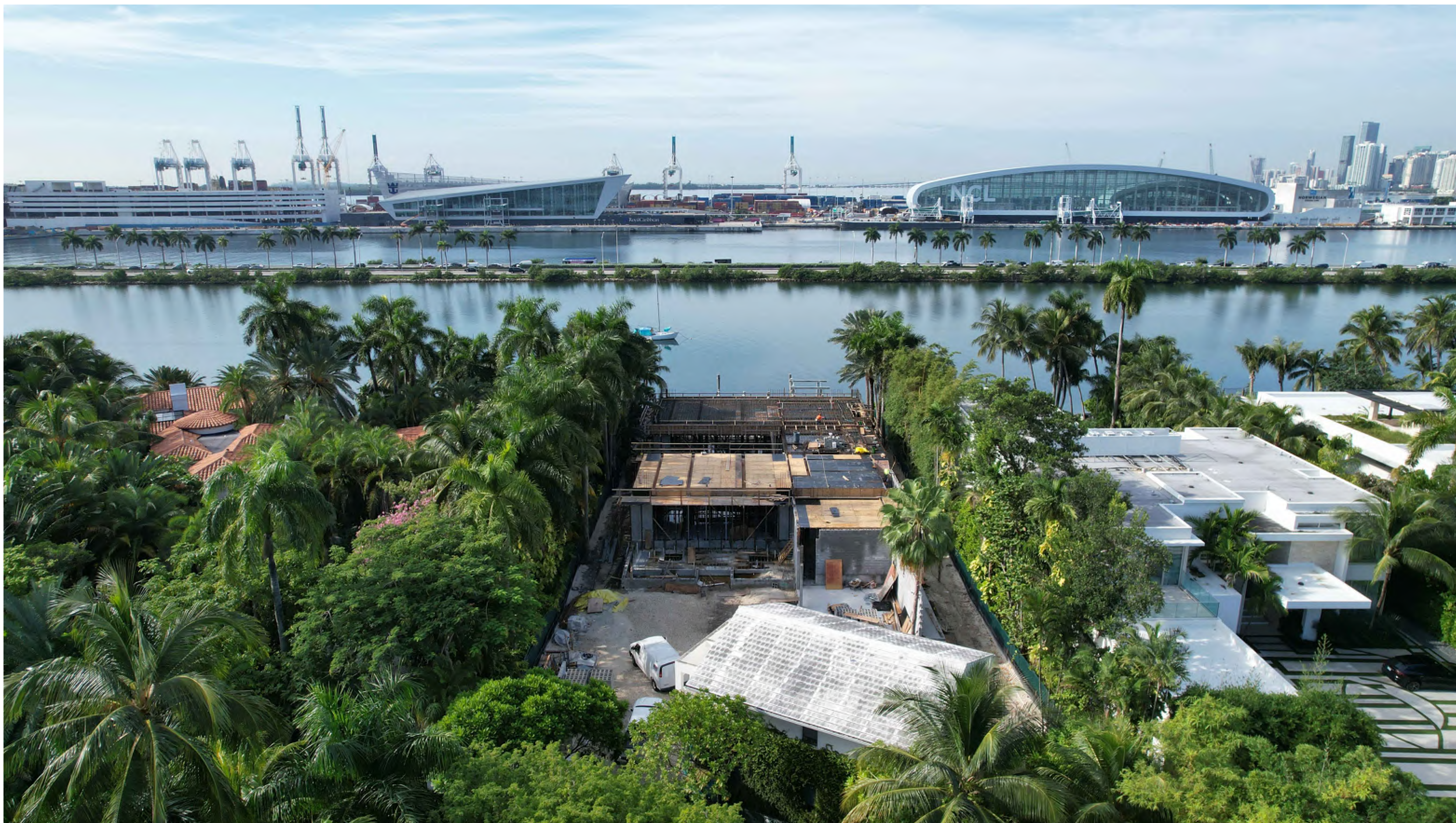
02 SOUTH VIEW - AERIAL SITE PHOTO (10/10/2023)
