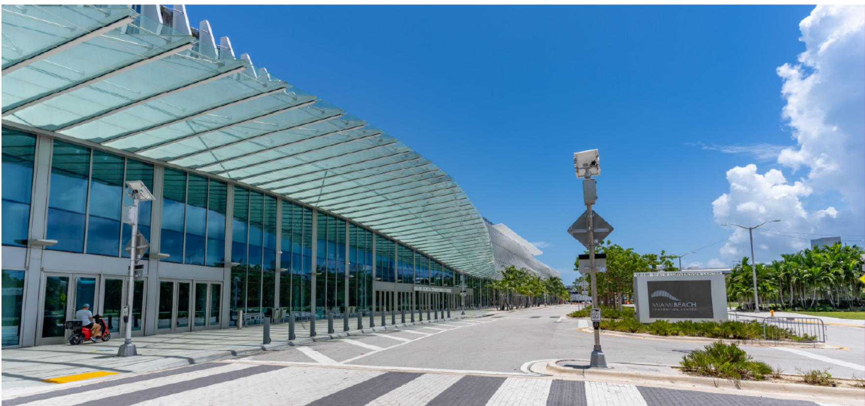
2. VIEW OF SITE FROM NORTHWEST
