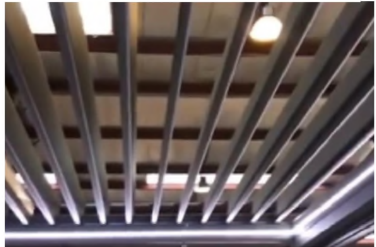
② RETRACTABLE LOUVERED SYSTEM INSTALLED IN DORAL CITY PLACE
