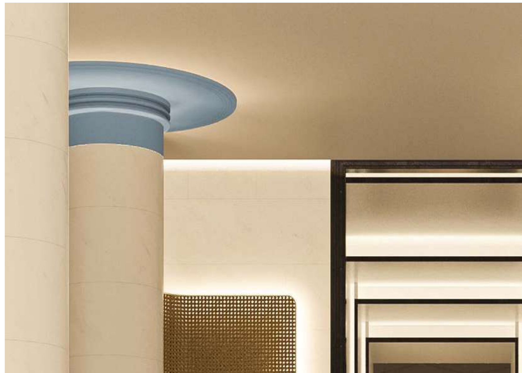
Cove lighting at perimeter interior walls
