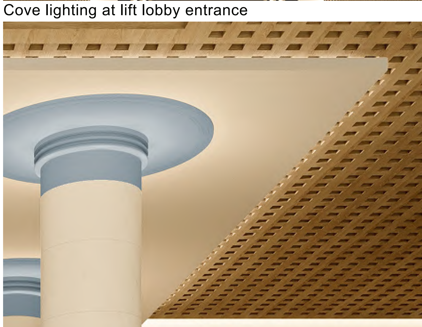
Cove lighting at drop ceiling
