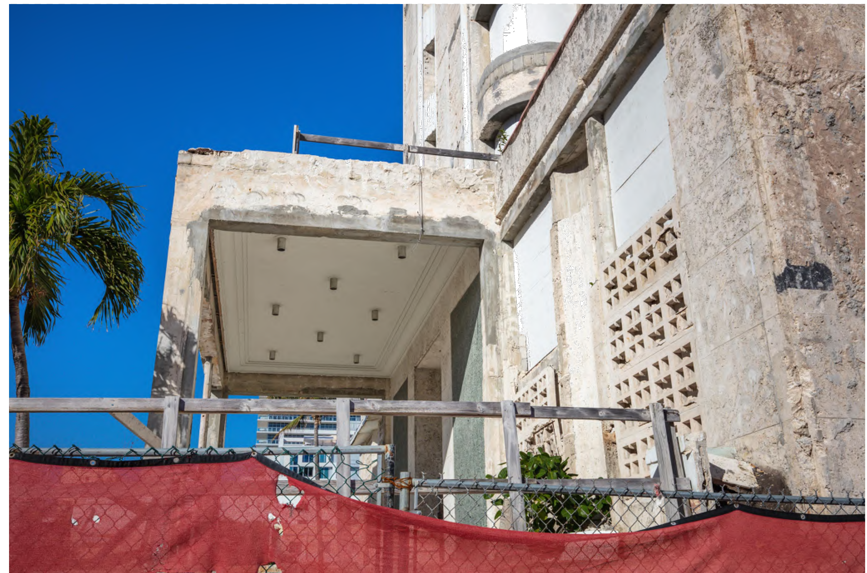
EXTERIOR - EXISTING CONDITIONS
