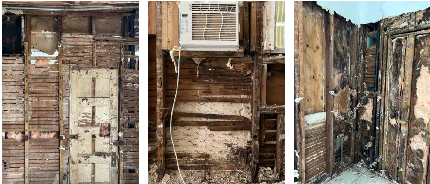
EXISTING INTERIOR CONDITIONS PHOTOS
