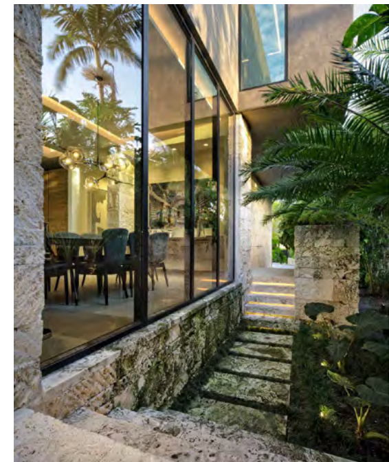
STONE TILE CLADDING
