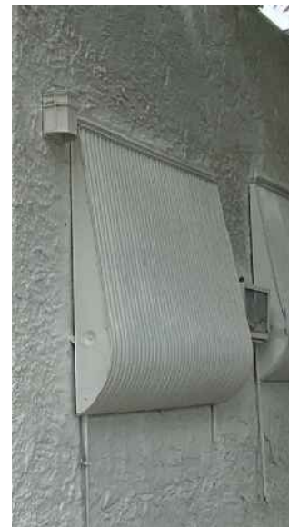
Aluminum fold down awnings installed in 1974 for privacy and solar protection
