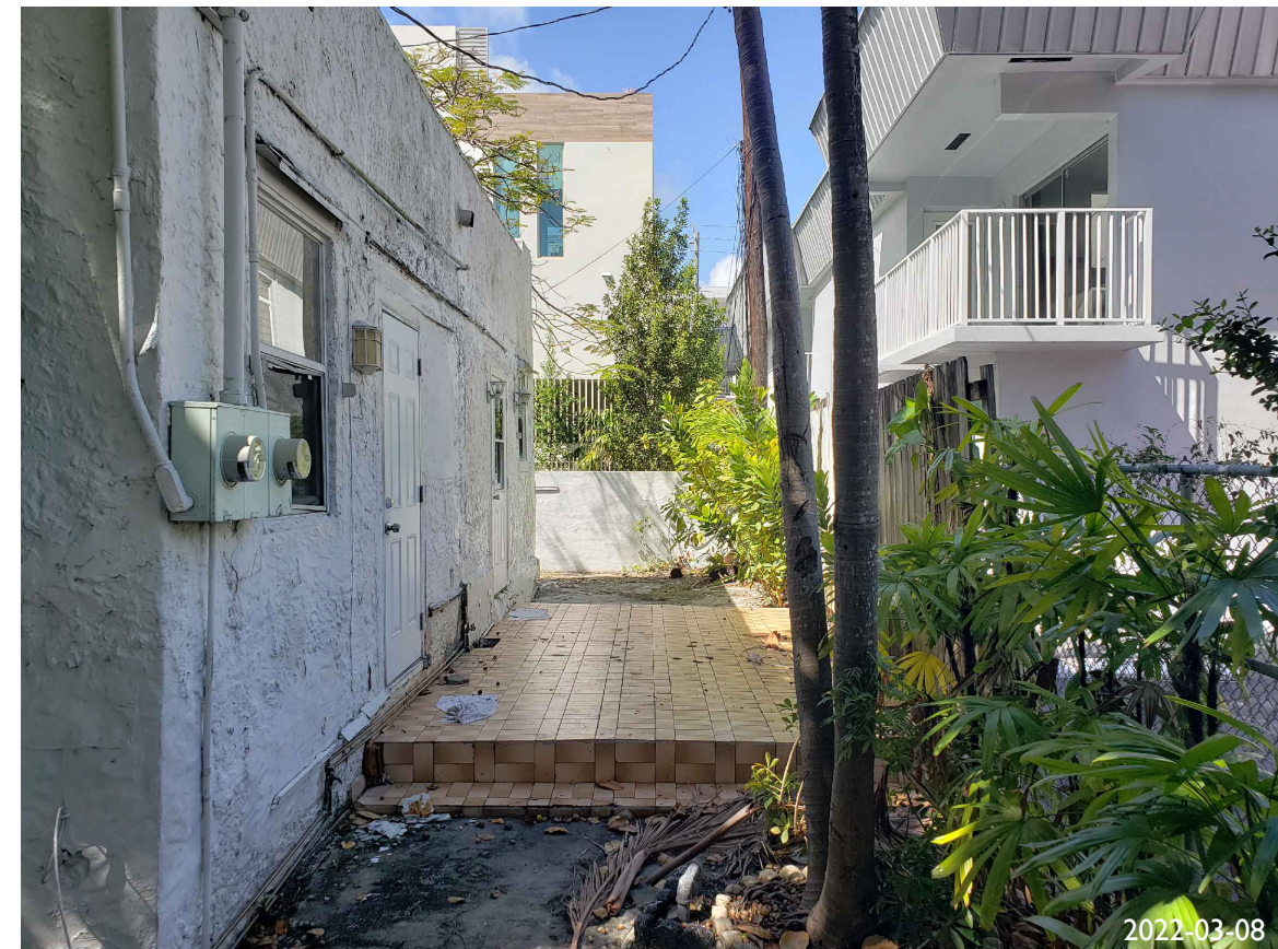
2. REAR DOORS OF EXISTING BUILDING
