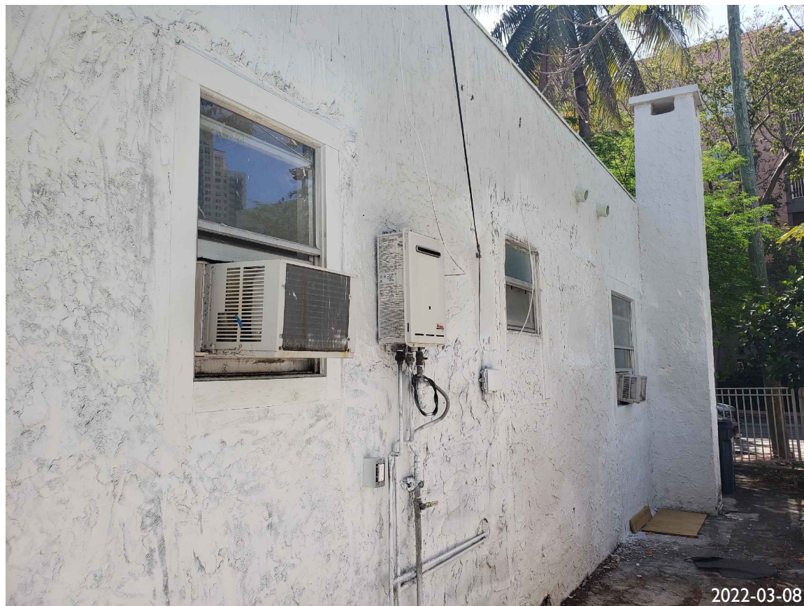
4. WEST FACADE OF EXISTING BUILDING
