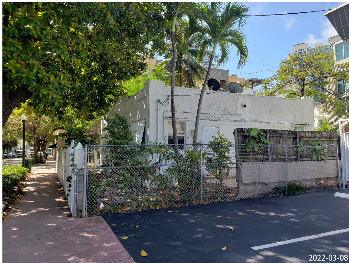
1. NORTH FACADE FACING RESIDENTIAL BUILDING AT 208 MERIDIAN
