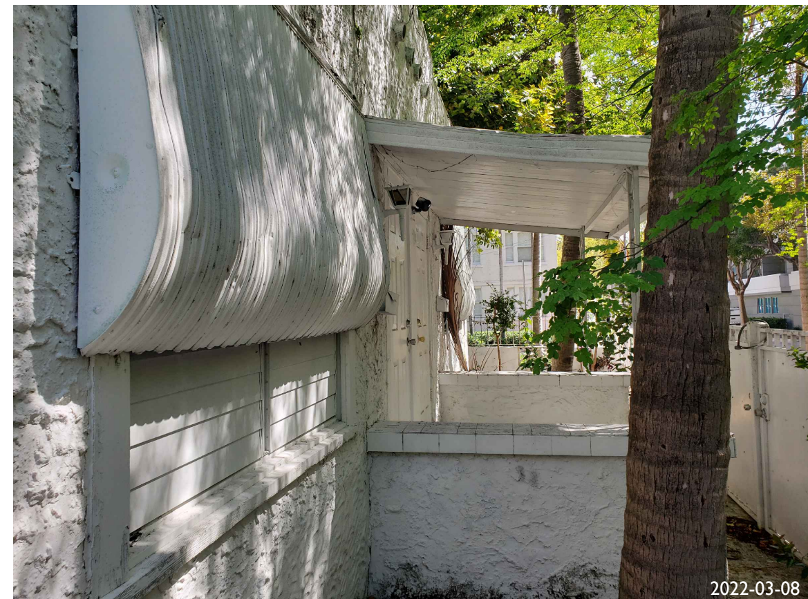
3. SOUTH FACADE FRONT ENTRANCE OF EXISTING BUILDING
