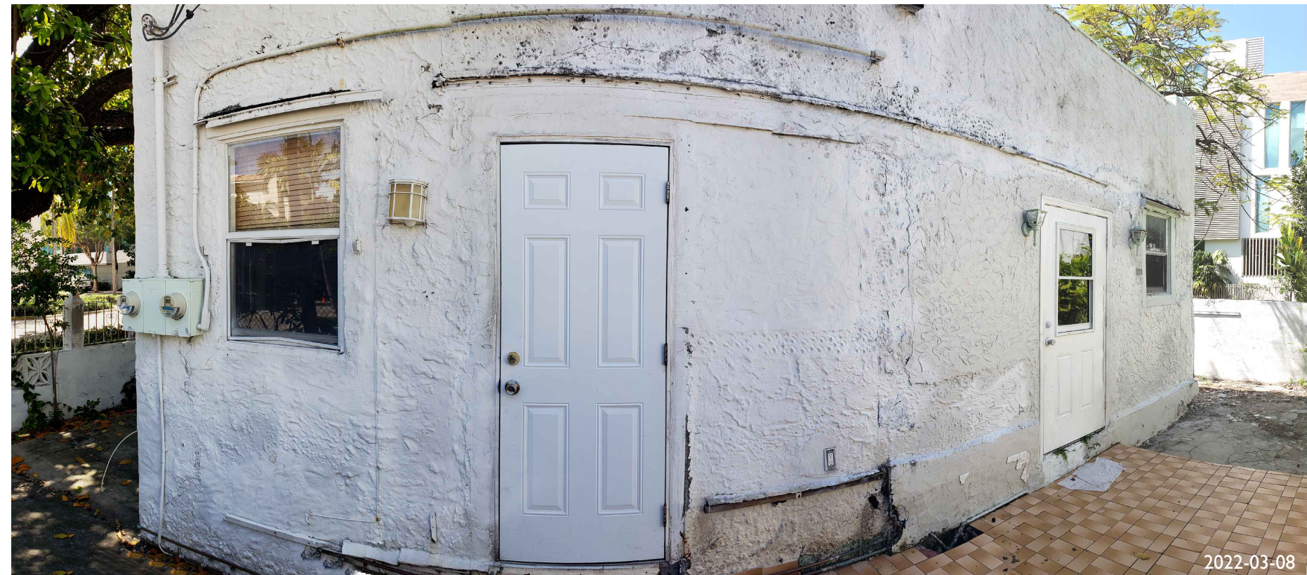
8. NORTH FACADE OF EXISTING BUILDING
