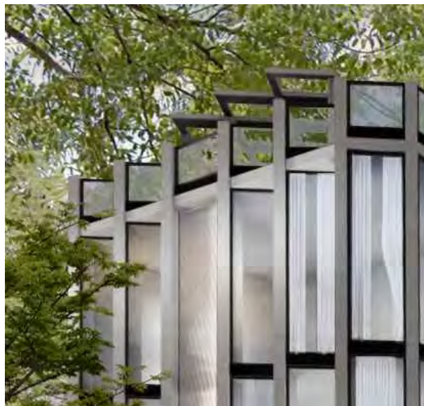
Faceted façade angled away from the adjacent buildings line of sight towards the east views facing street intersection. Such orientation offers solar control and better views.
