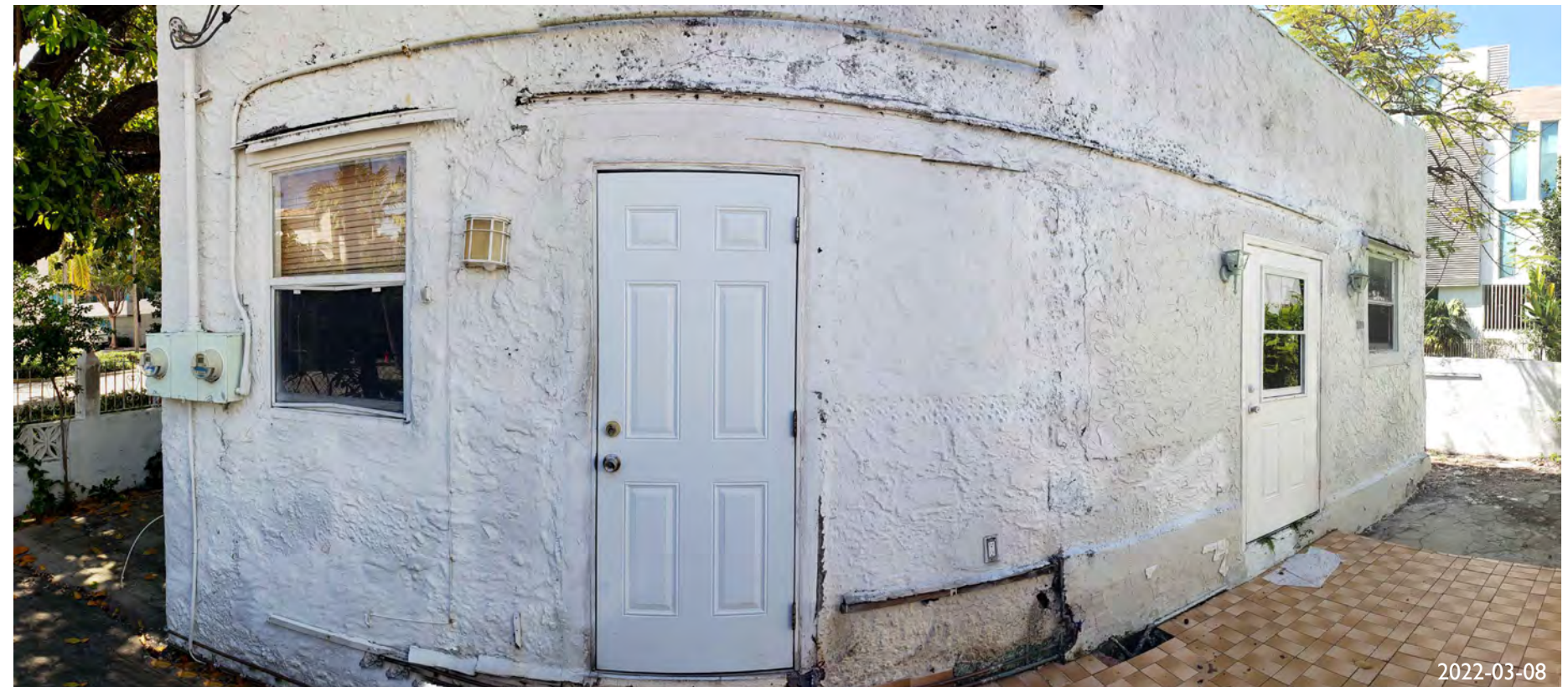
8. NORTH FACADE OF EXISTING BUILDING
