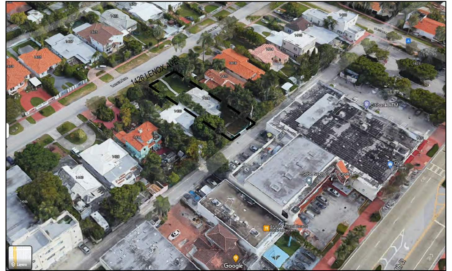
2 REAR AERIAL VIEW
