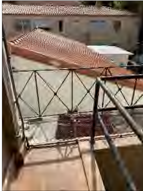
VIEW 5 BALCONY EAST VIEW
