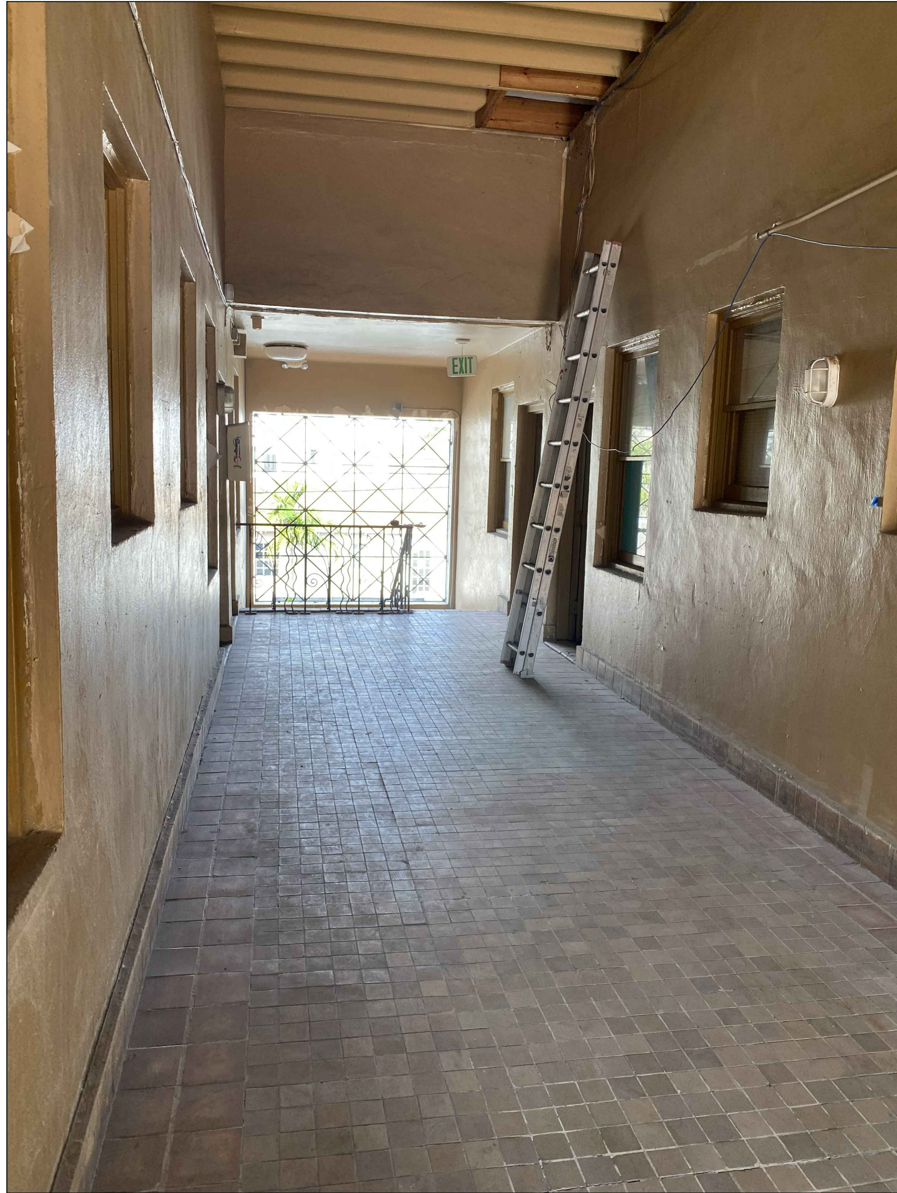
VIEW 1 CORRIDOR WEST VIEW
